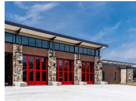
GRAPEVINE, TX FIRE STATION NO. 2
