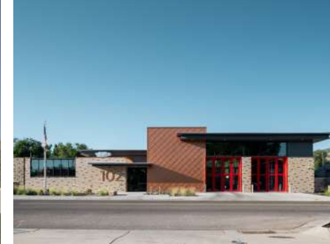
UFA FIRE STATION NO 102 | MAGNA, UT
