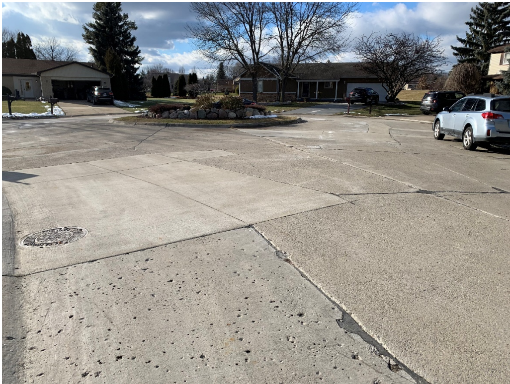
Mill Road Court West (Whispering Meadows Sub) – Large panel replacements
