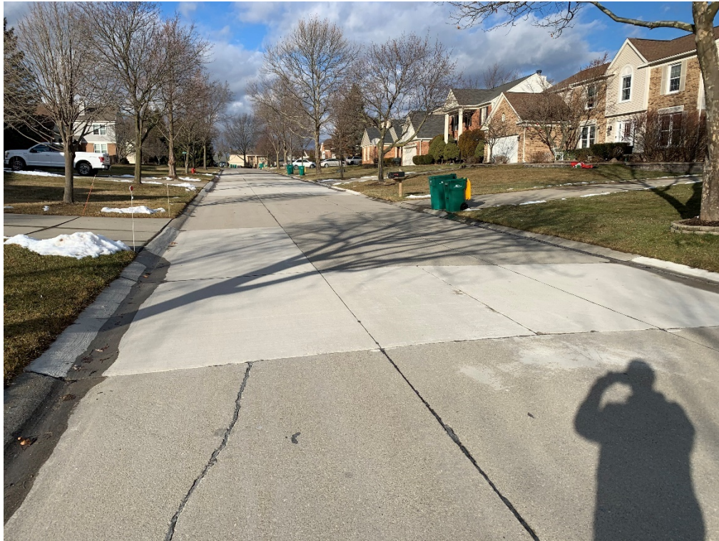
Waycroft Drive (Dunbarton Pines Sub) – Intermixed panel replacements
