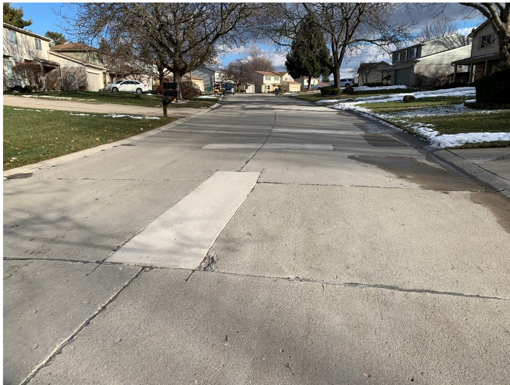
Mill Road (Whispering Meadows Sub) – Discrete panel replacements
