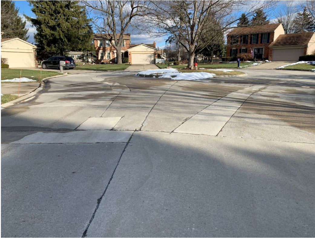
Mill Road Court East (Whispering Meadows Sub) – Centerline panel replacements
