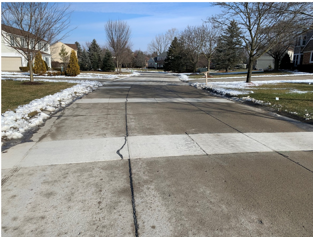
Daleview Drive (Lexington Green Sub) – Full width panel replacements
