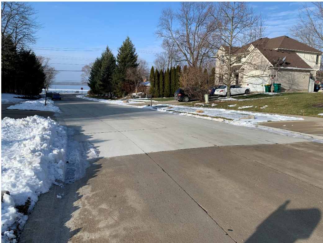
Morgan Creek Court (Morgan Creek Sub) – Full width replacement
