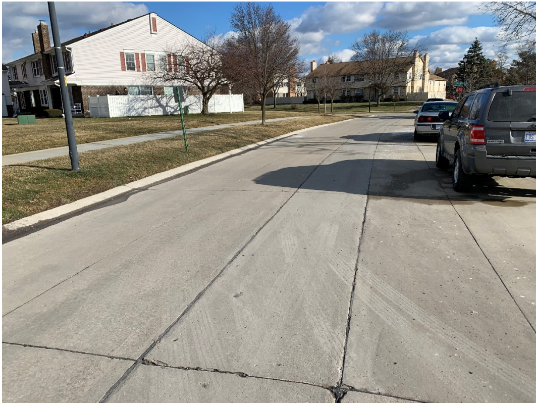
Pellston Drive (Country Place Condominiums) – Center line panel replacements
