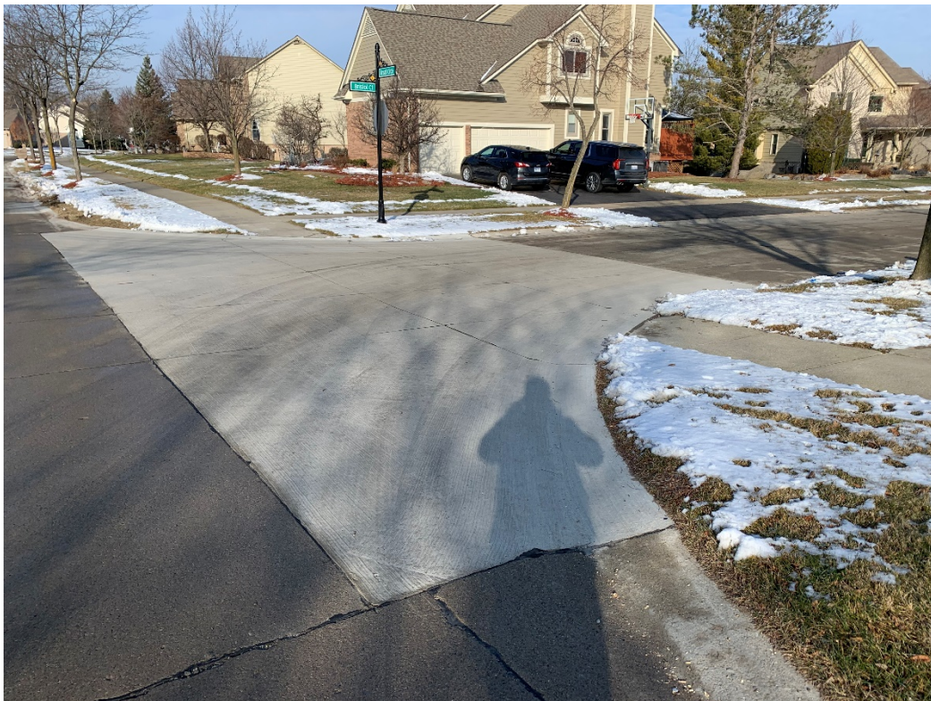
Balfour Drive and Court (Bristol Corners West Sub) – Full width panel replacements
