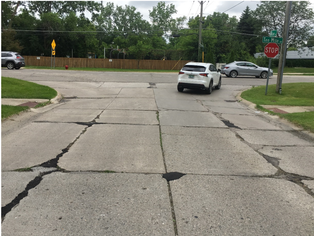
Nilan Drive (Fairfield Farms Sub) @ 10 Mile – Pre-Construction
