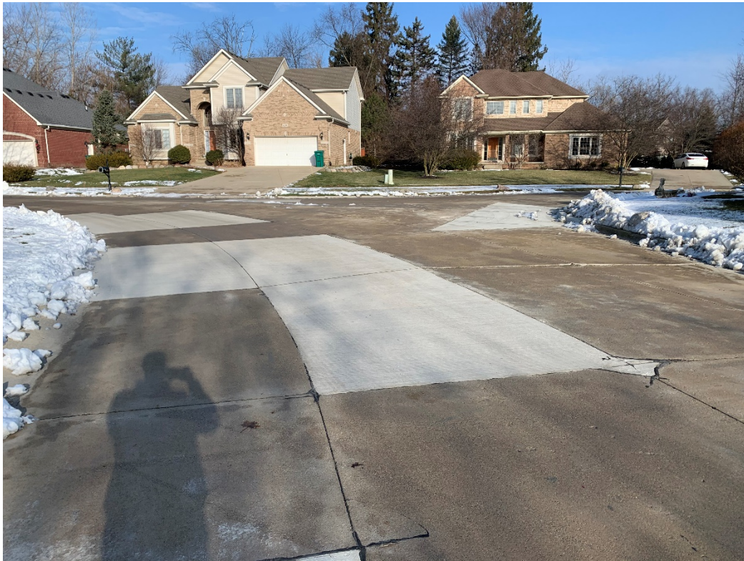
Morgan Creek Court (Morgan Creek Sub) – Discrete panel replacements in cul-de-sac
