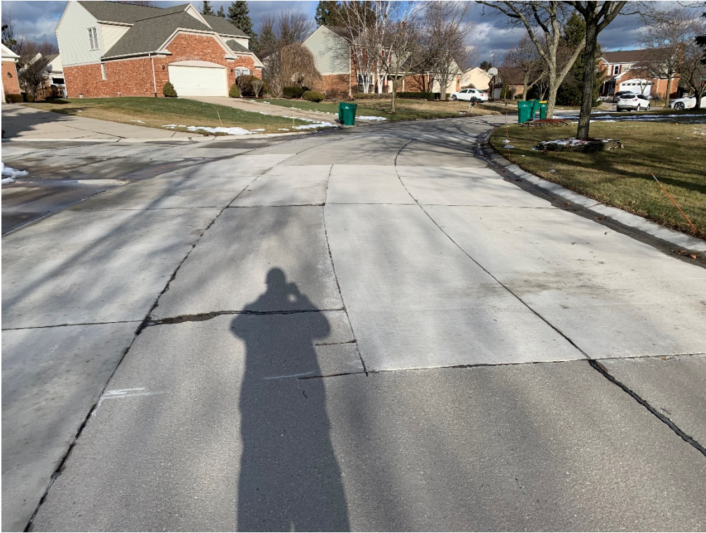
Courtview Trail (Dunbarton Pines Sub) – Intermixed panel replacements
