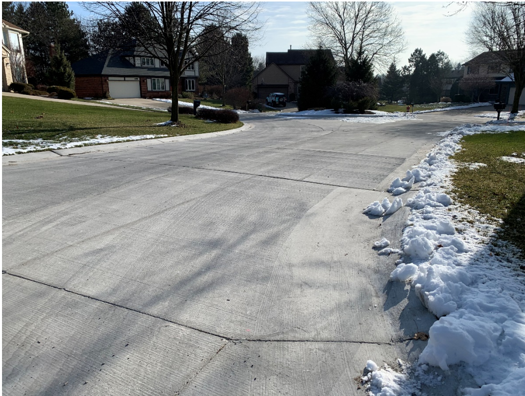
Dunbarton Court (Dunbarton Pines Sub) – Complete concrete replacement
