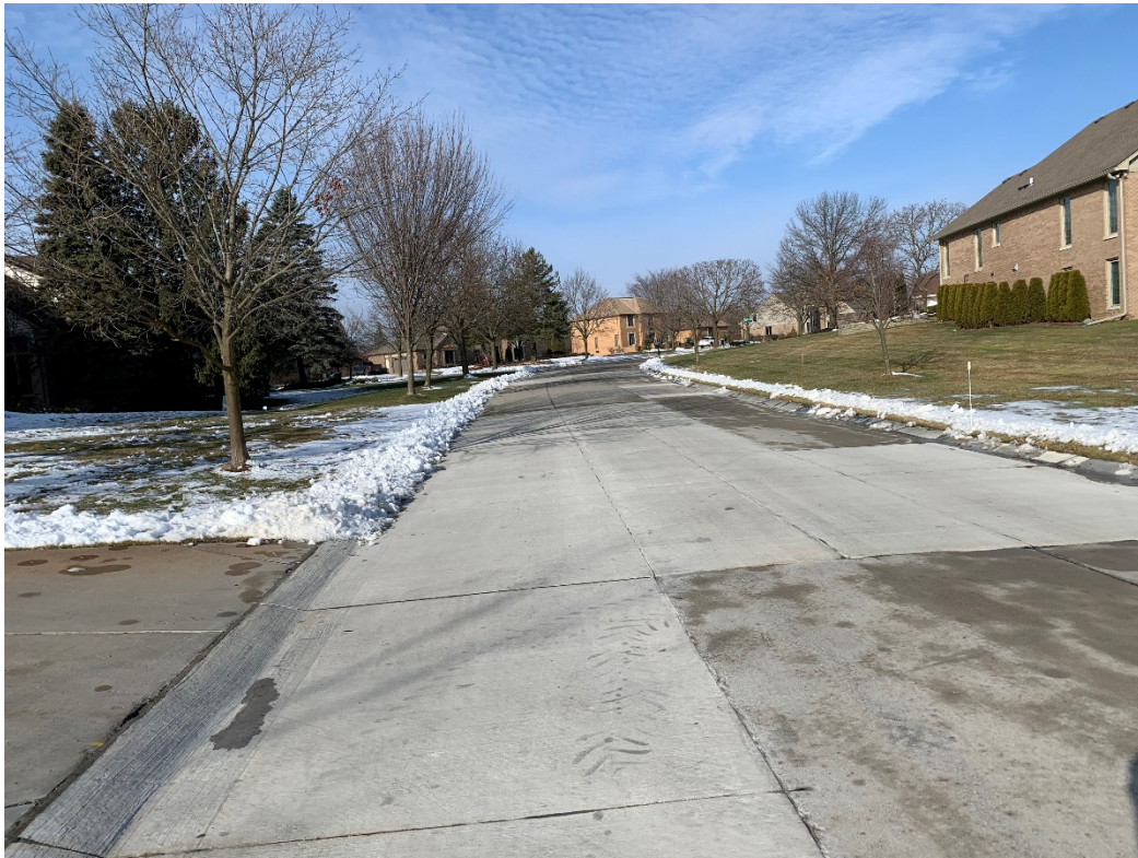
Daleview Drive (Lexington Green Sub) – Large panel replacements
