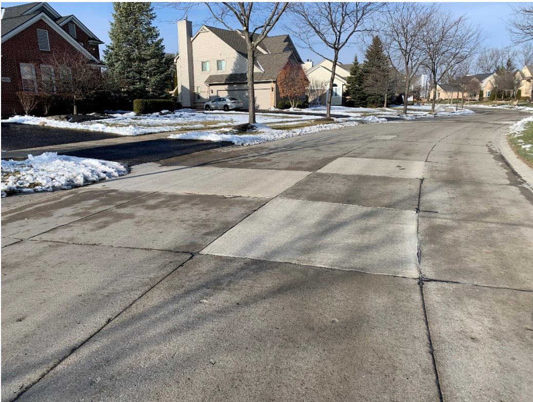
Bristol Circle West (Bristol Corners West Sub) – Discrete individual panels
