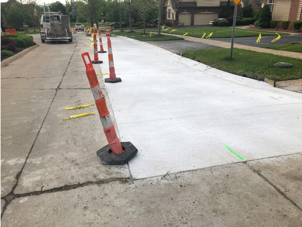
Bristol Circle Court (Bristol Corners West Sub) – Large patch (1 st half)
