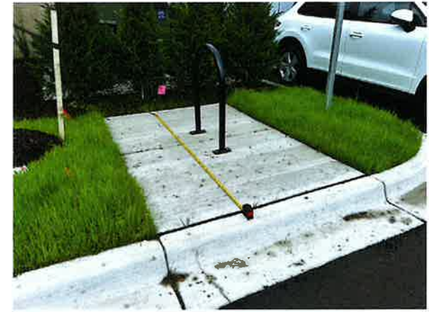
FIGURE 4: During site inspections, AECOM verifies the placement and dimensions of signing, pavement markings, and other traffic related components.
