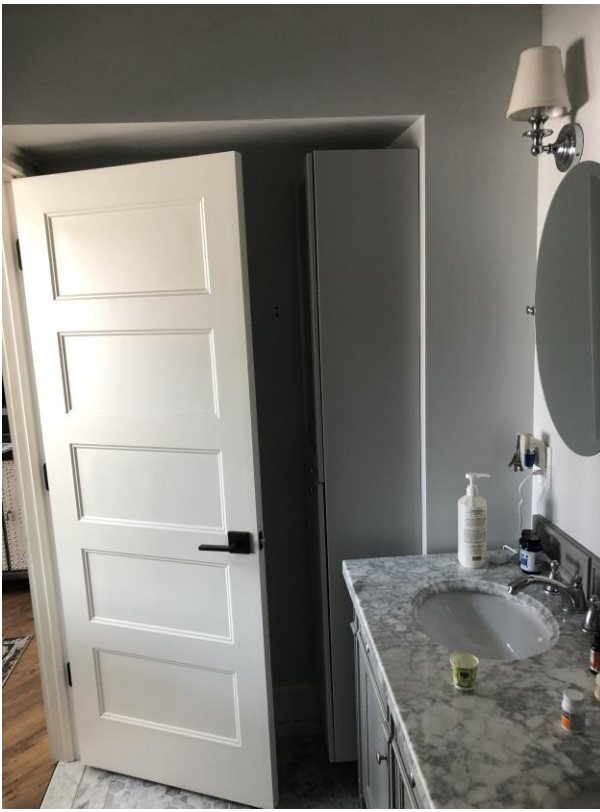
EXISTING MASTER BATHROOM IS 5' WIDE WITH POOR FUNCTIONALITY.
