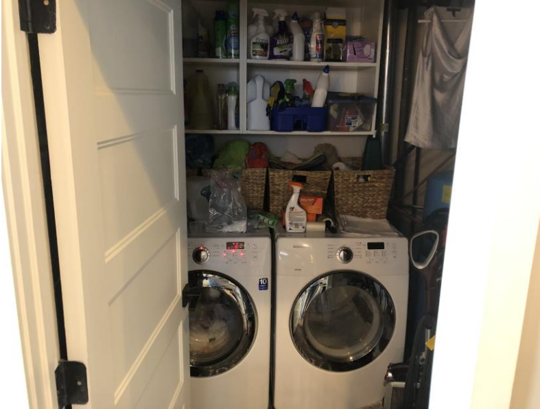
EXISTING FIRST FLOOR CENTRALLY LOCATED MECHANICAL ROOM IS SLAB ON GRADE AND FURNACE AND WATER TANKS HAVE LIMITED ACCESSIBILITY WITH LAUNDRY MACHINES IN THE SAME ROOM.
