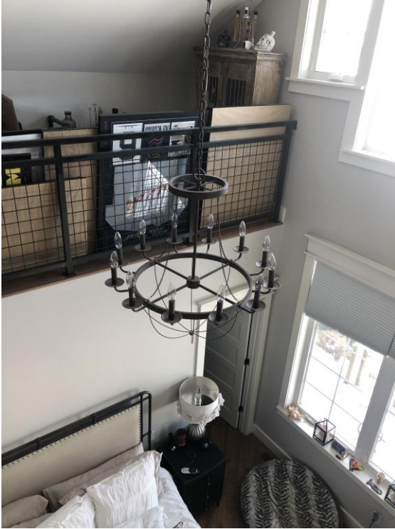
UNUSABLE PRE-EXISTING CONDITIONS IN ATTIC LEVEL.
