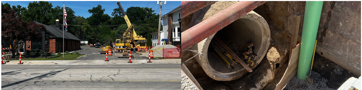
CENTER STREET WORKSITE
