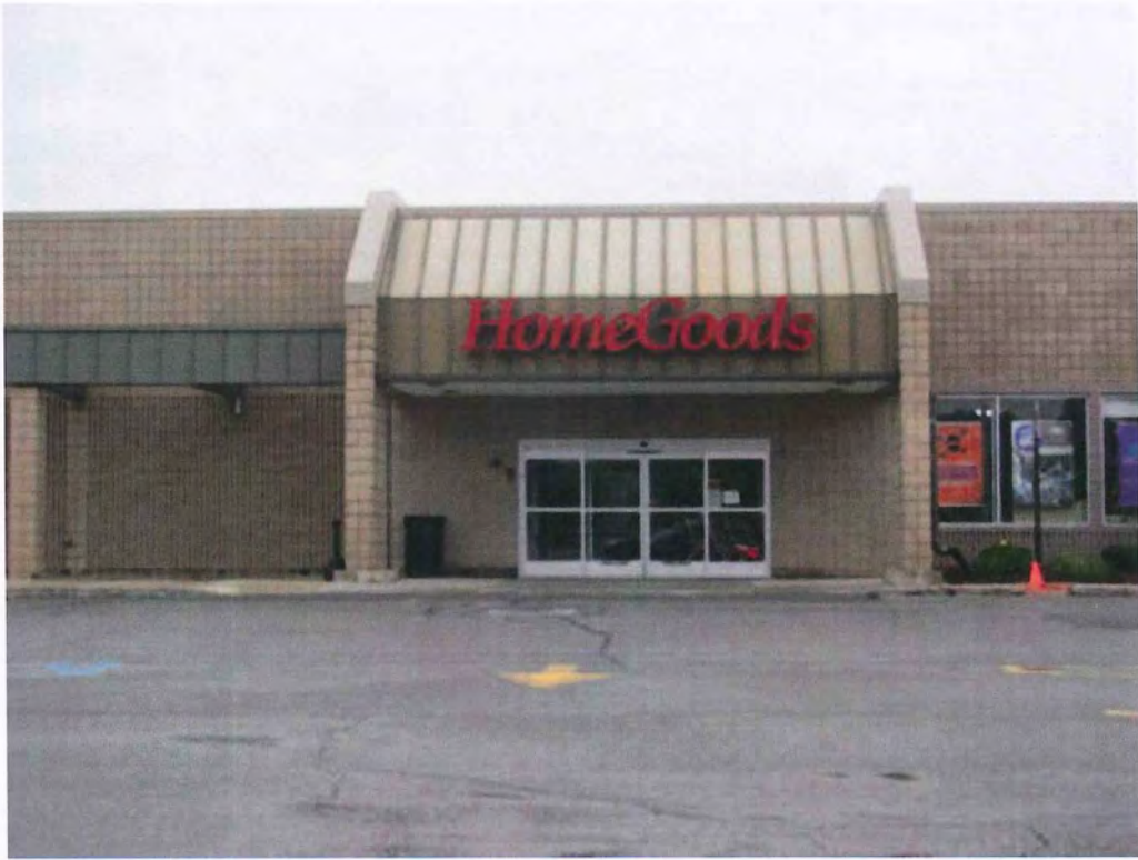
Existing Home Goods entrance
