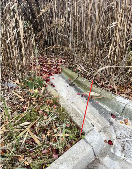
PP 7, Outfall from Parking Lot
