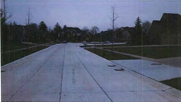
Full concrete reconstruction of Dukesbury Ct.
