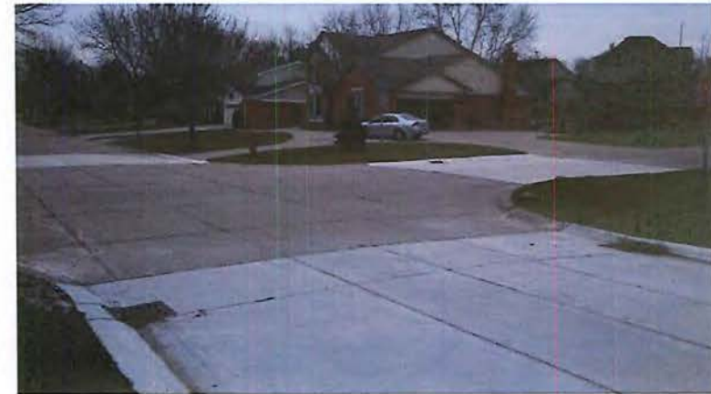
Slab replacement at Foxton/Huntingcross Drives
