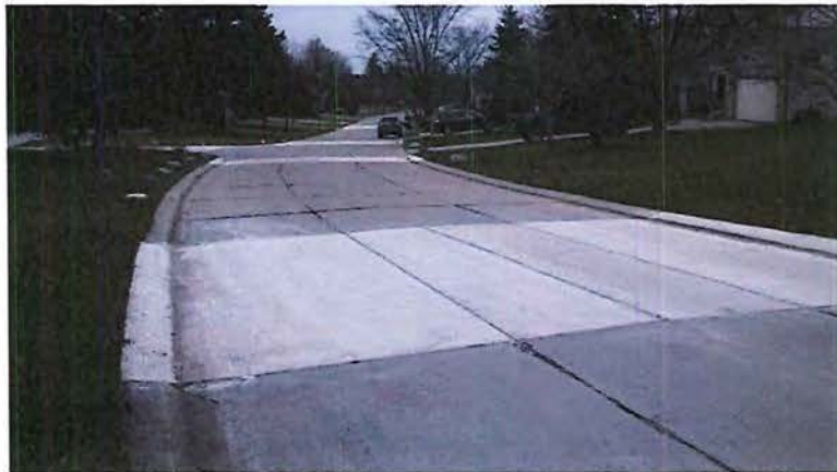
Panel joint/slab replacement on Dunbarton Drive
