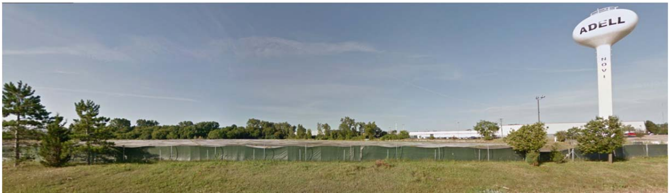
Existing Streetscape along I-96 frontage
