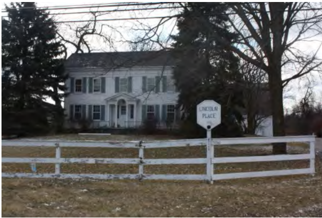
Lincoln Place, 47133 West Nine Mile (ca 1838)
