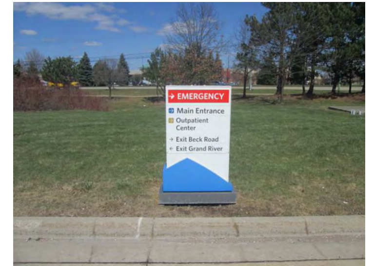
Existing 4'-10" x 2'-6" signage to be removed & replaced; Install far enough away to avoid existing footer
