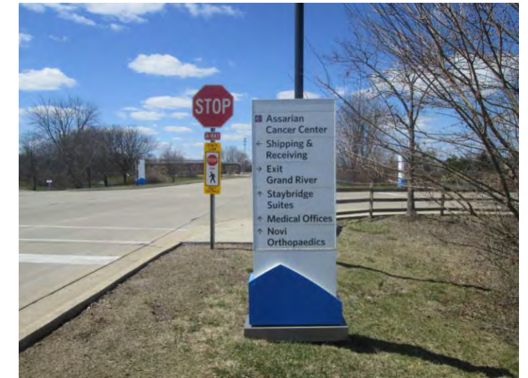
Existing 6'-6" x 2'-6" signage to be removed & replaced; Installed far enough away to avoid existing footer
