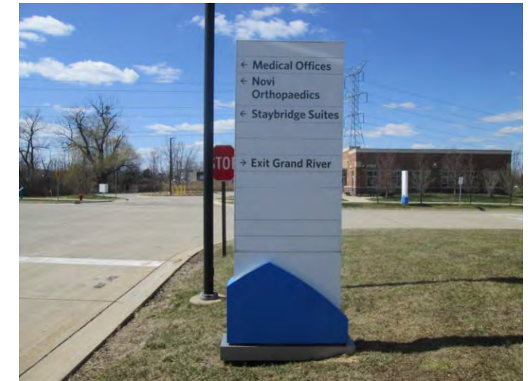
Existing 9'-10" x 3'-4" signage to be removed & replaced; Install far enough away to avoid existing footer
