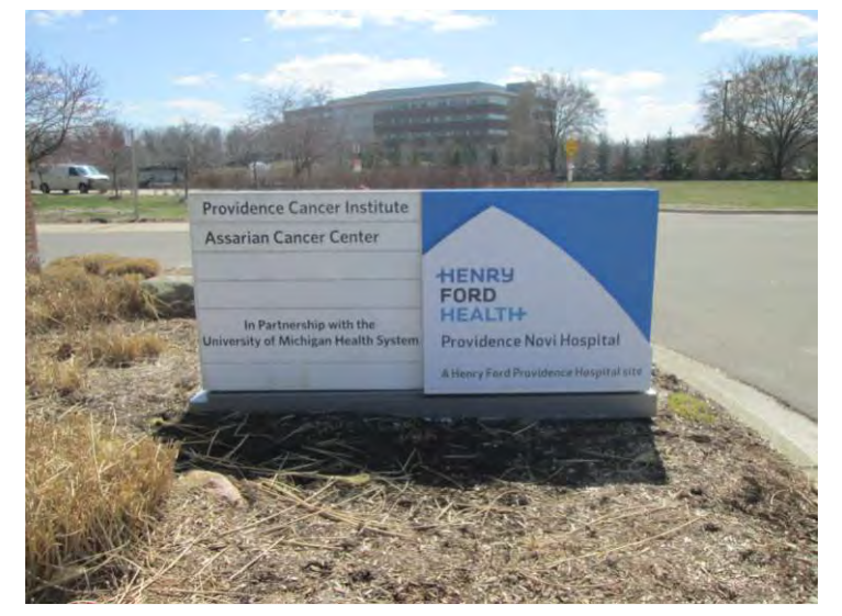
Existing 4'-0" x 8'-0" signage to be removed & replaced; Install far enough away to avoid existing footer
