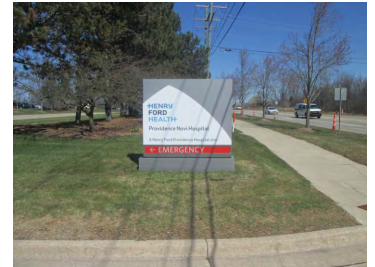
Existing 5'-10" x 6'-6" signage to be removed & replaced; Install far enough away to avoid existing footer
