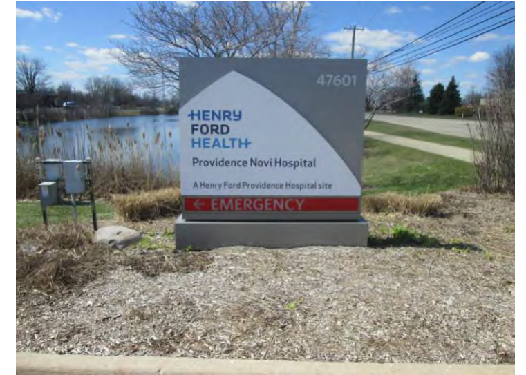
Existing 5'-10" x 6'-6" signage to be removed & replaced; Install far enough away to avoid existing footer
