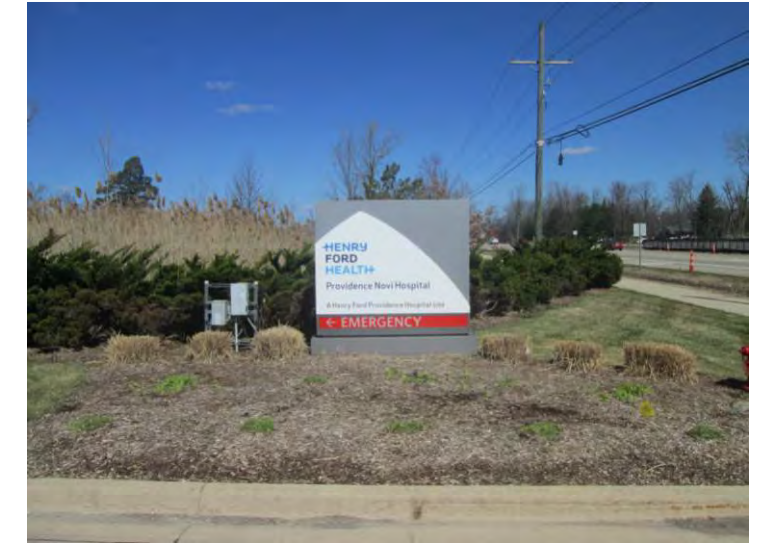
Existing 5'-10" x 6'-6" signage to be removed & replaced; Install far enough away to avoid existing footer
