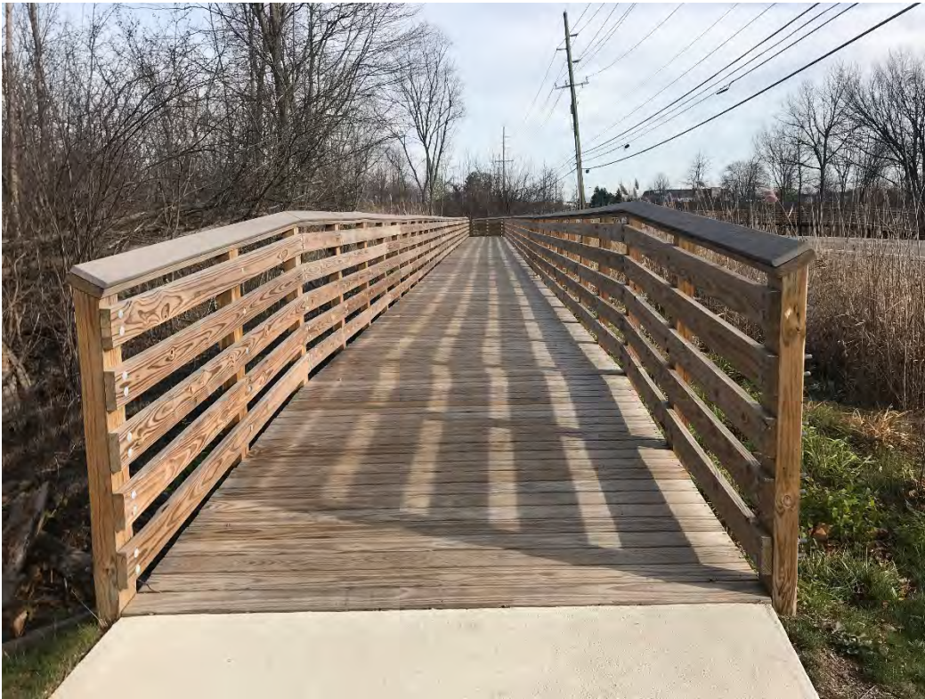
Boardwalk No. 5 – North-side of 10 Mile, just east of Churchill Boulevard
