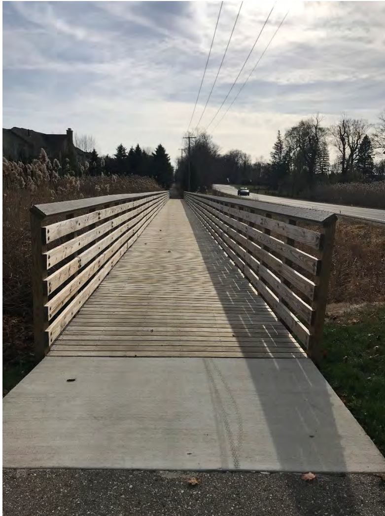
Boardwalk No. 33 – East-side of Napier Road, just south of Seaglen Drive
