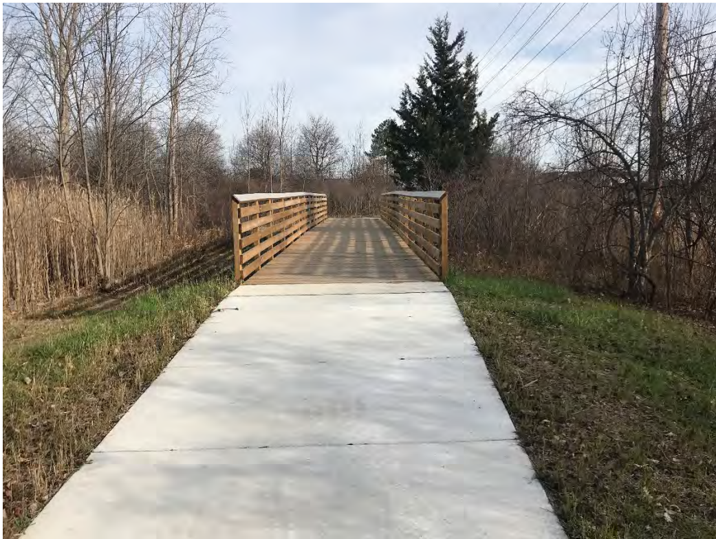
Boardwalk No. 4 – North-side of 10 Mile, just west of Novi Road
