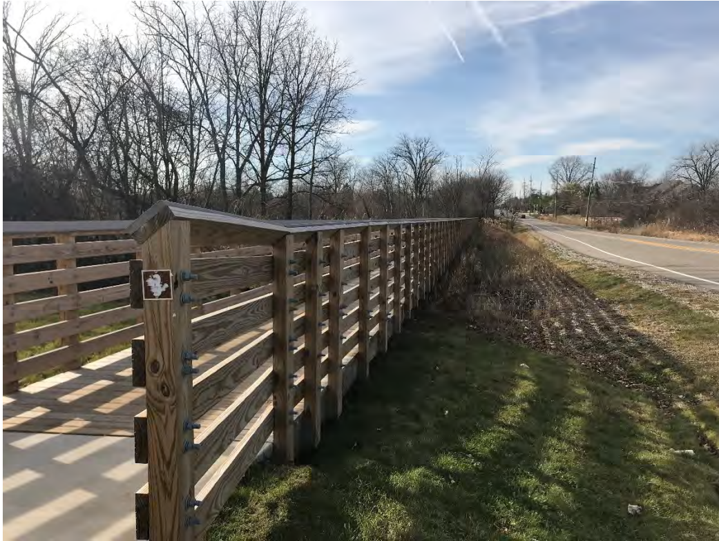
Boardwalk No. 3 – South-side of 10 Mile between Senior Center and Cortland Boulevard
