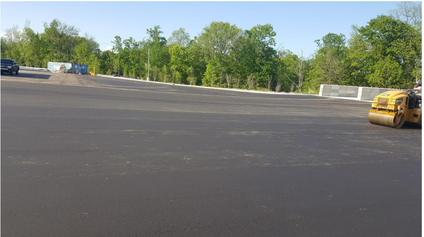
DPW (east lot) – Finish rolling the final lift of asphalt
