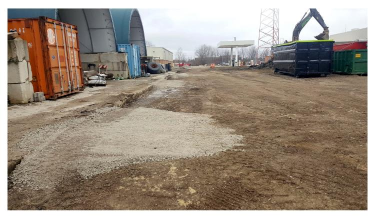
DPW South Lot, Auxiliary Storage Domes and Fuel Station – Excavation of existing asphalt
