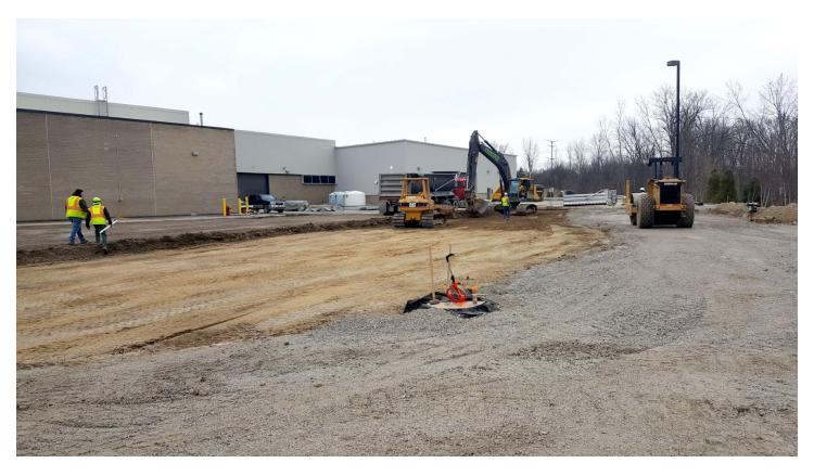
DPW (main building and east lot) - Existing asphalt lot excavation, compaction and stone placement
