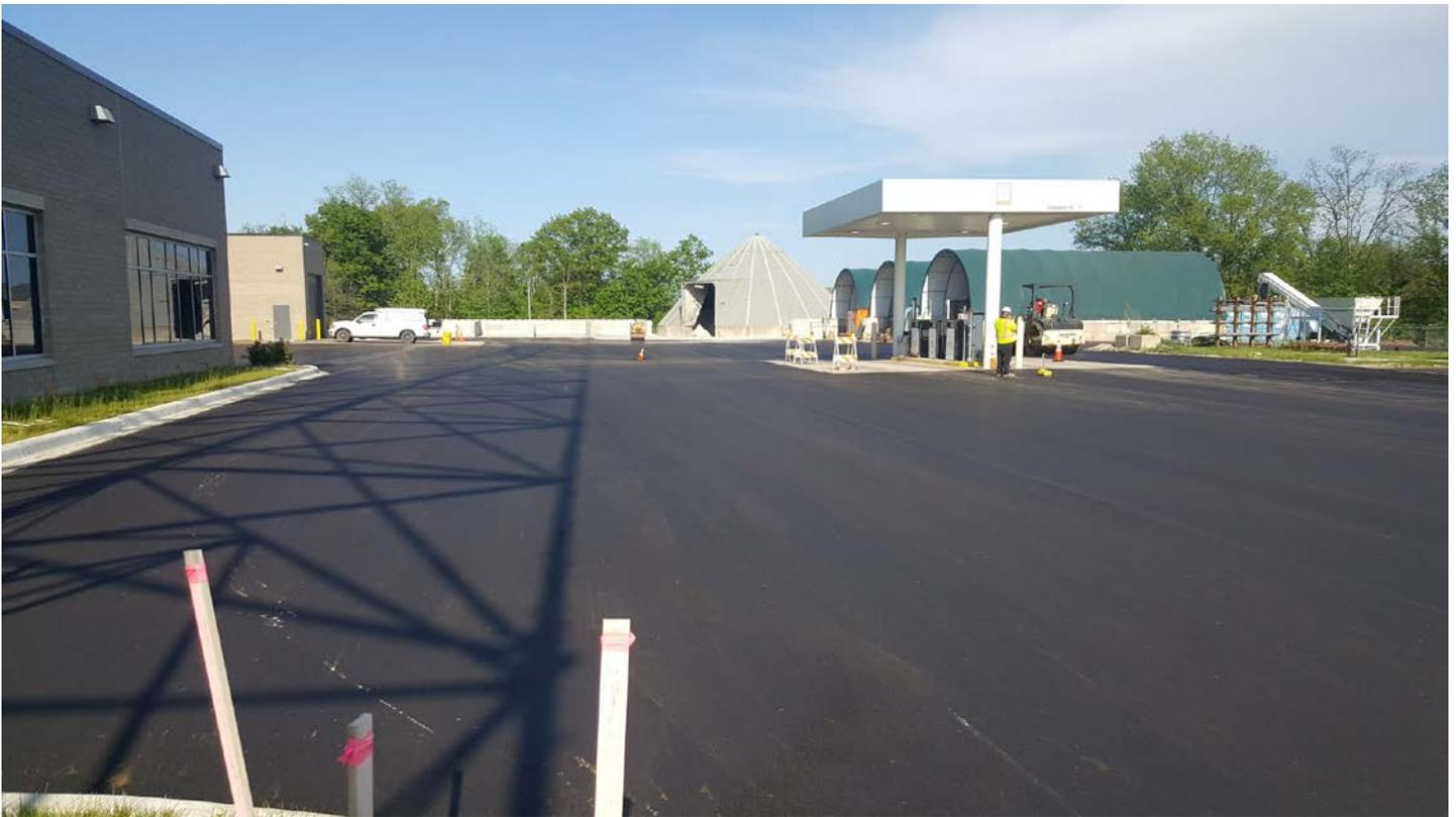
DPW South Lot, Main Building and Fuel Station – Finish rolling of the final asphalt lift
