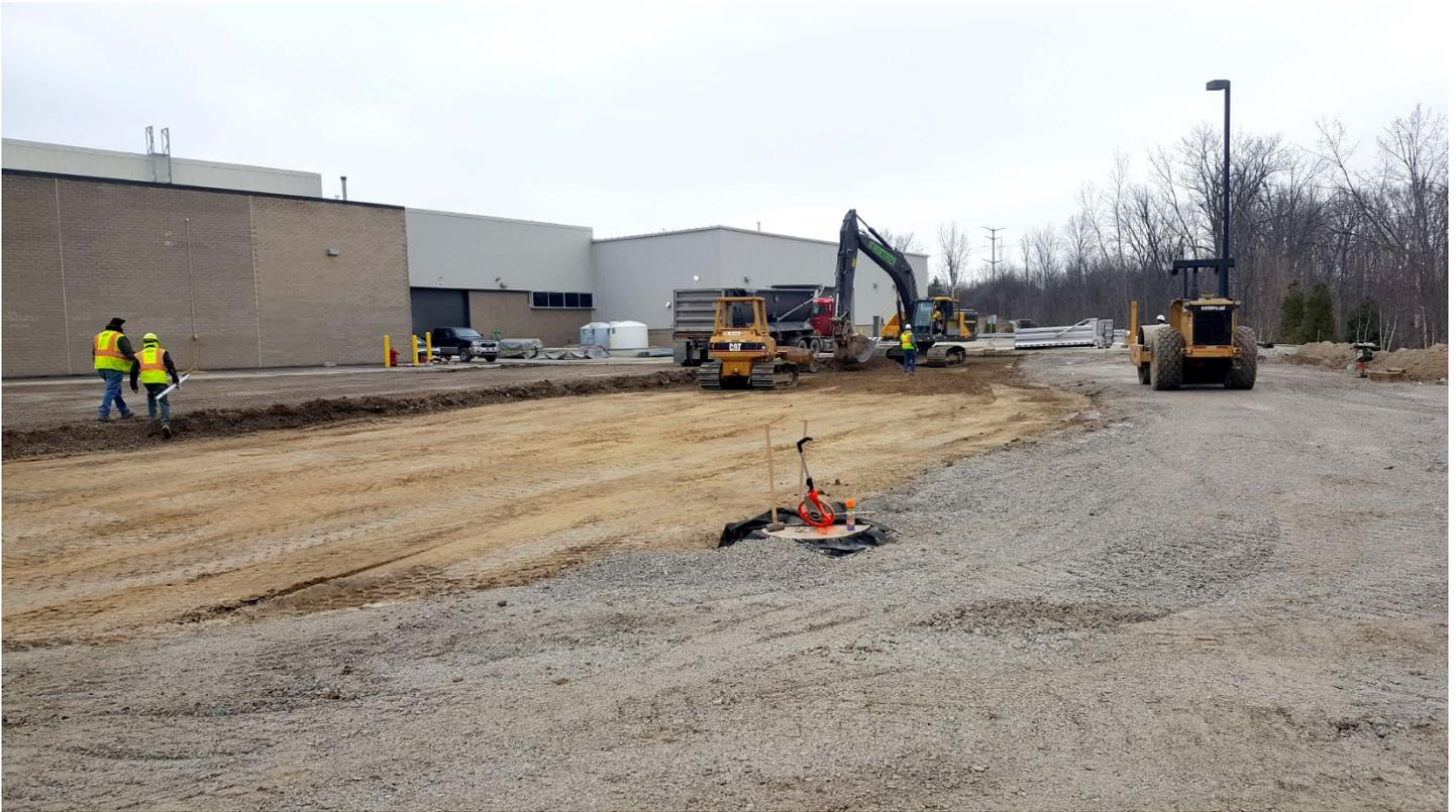
DPW (main building and east lot) – Existing asphalt lot excavation, compaction and stone placement
