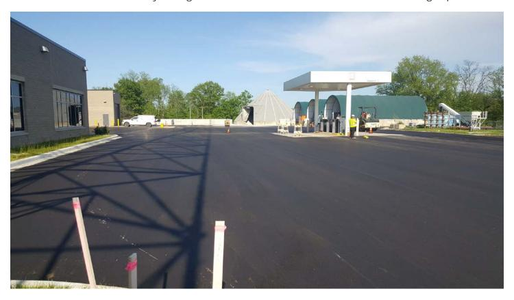
DPW South Lot, Main Building and Fuel Station – Finish rolling of the final asphalt lift
