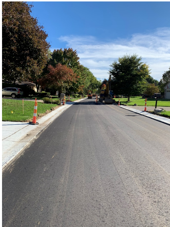
Siegal Court (Turtle Creek Sub) – Singh Boulevard to the cul-de-sac (First lift)
