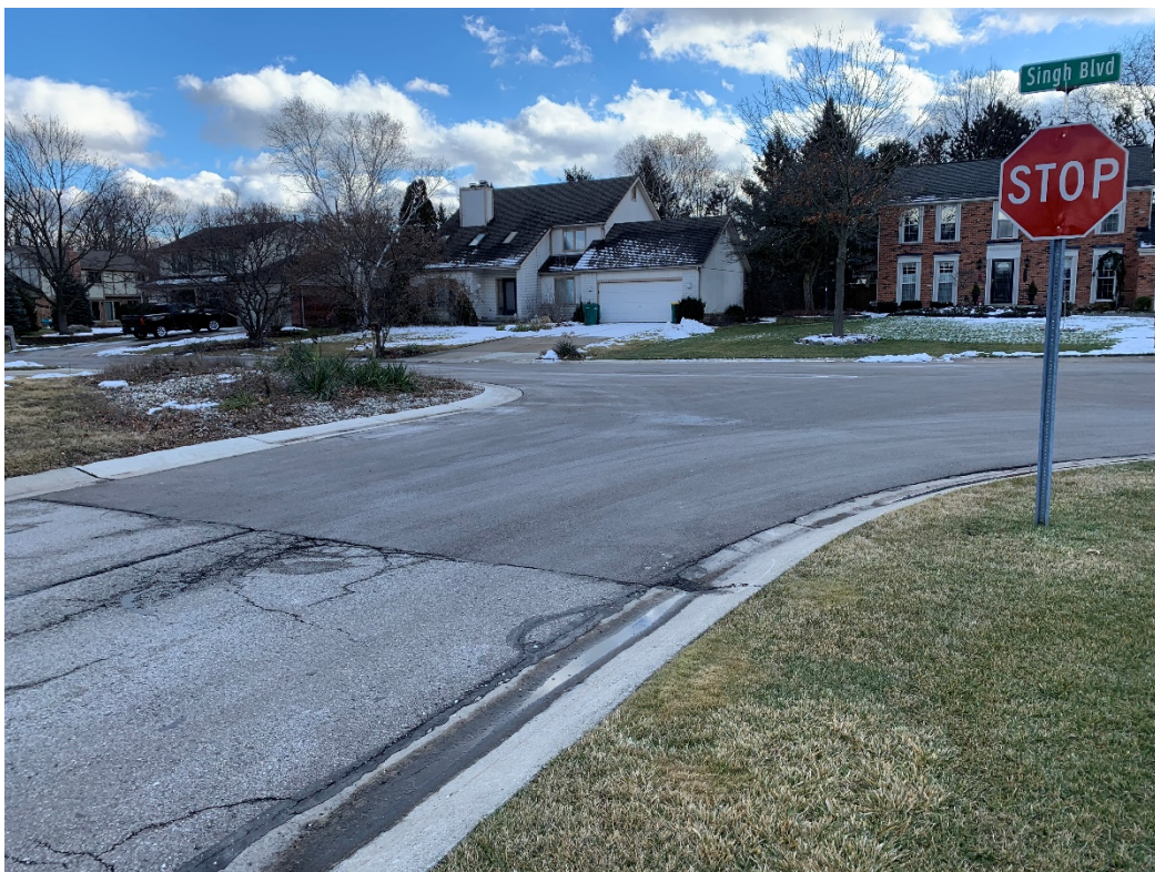
Singh Boulevard (Turtle Creek Sub) – at Cascade Drive looking south
