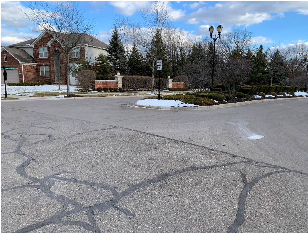
Churchill Boulevard (Churchill Crossing Sub) – Entranceway from Cavendish Ave
