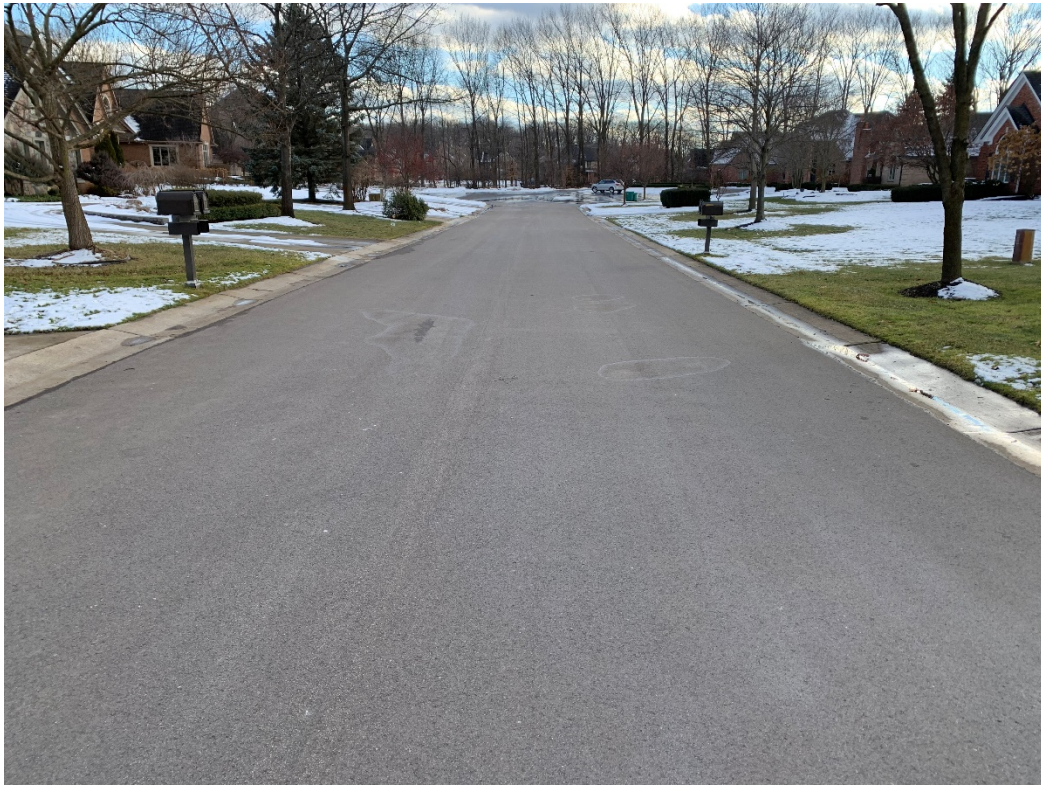
Vero Court (Vero Sub) – Looking west from Novi Road
