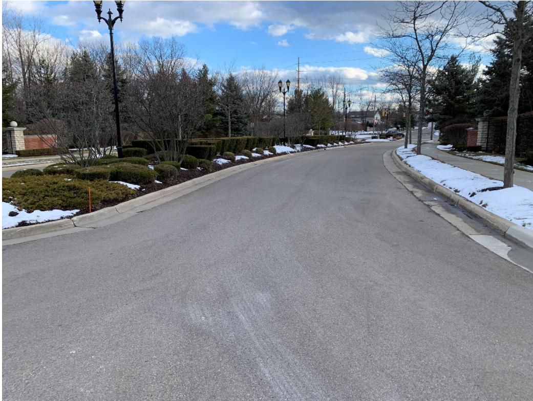
Churchill Boulevard (Churchill Crossing Sub) – Entranceway from 10 Mile
