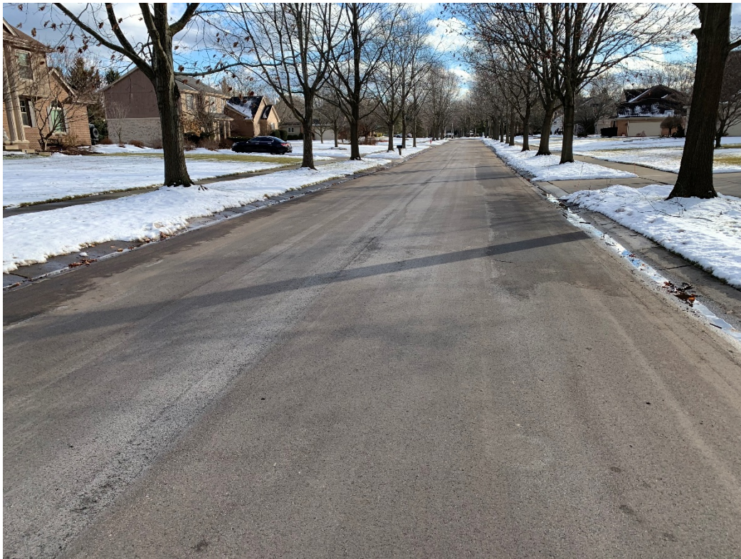
Lynwood Drive (Greenwood Oaks Sub) – Looking north from Warrington Drive
