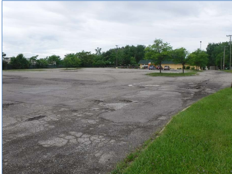
Photo 1. View of the existing DICE building from near Novi Road (ECT, June 19, 2018).
