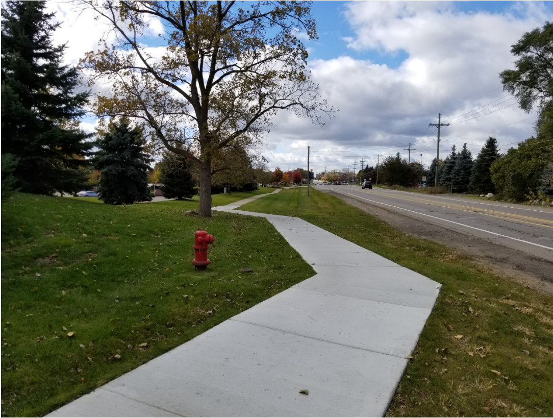
West end tie-in to existing sidewalk at Portsmouth Apts. and Kroger.
