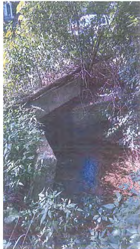
East End of Bridge
