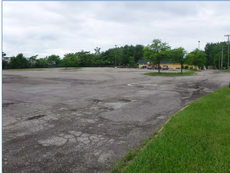
Photo 1. View of the existing DICE building from near Novi Road (ECT, June 19, 2018).
