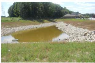
Additionally, modifications were made to the basin to improve the storm water quality treatment capabilities prior to discharging into the adjacent Zander Drain. The basin was retrofitted with an outlet control structure, a permanent water elevation, and native plantings to meet the minimum treatment requirements outlined in the Macomb County Public Works Procedures and Design Standards for Stormwater Management.
