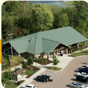
Lakeshore Park Building & Renovations
