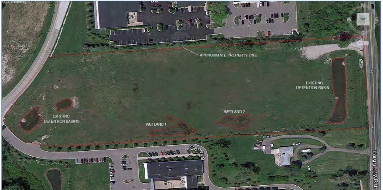
Figure 1. Aerial photo of the 29293 Haggerty Road Property. Existing non-essential wetland areas (Wetlands 1 and 2) and detention basins are indicated in red.
