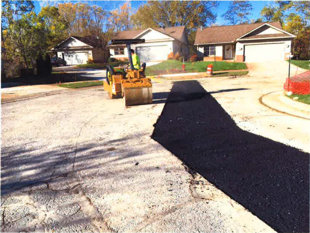
Placing new asphalt in the water main trench
