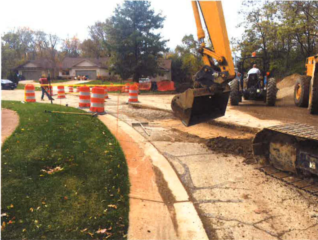
Backfilling the new water main within the Andes Hills Court cul-de-sac
