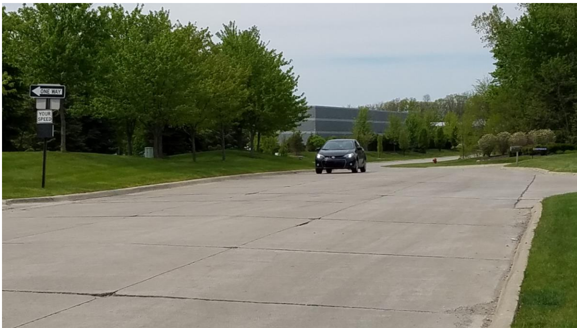
Figure 1. Northbound Radar Speed Sign Across from Peary Drive
