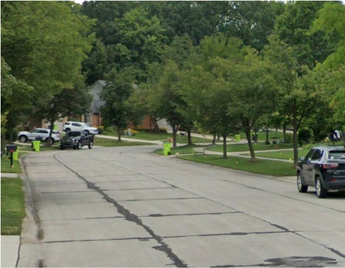
Before: White Pines Drive, looking north from Bertram Drive.
