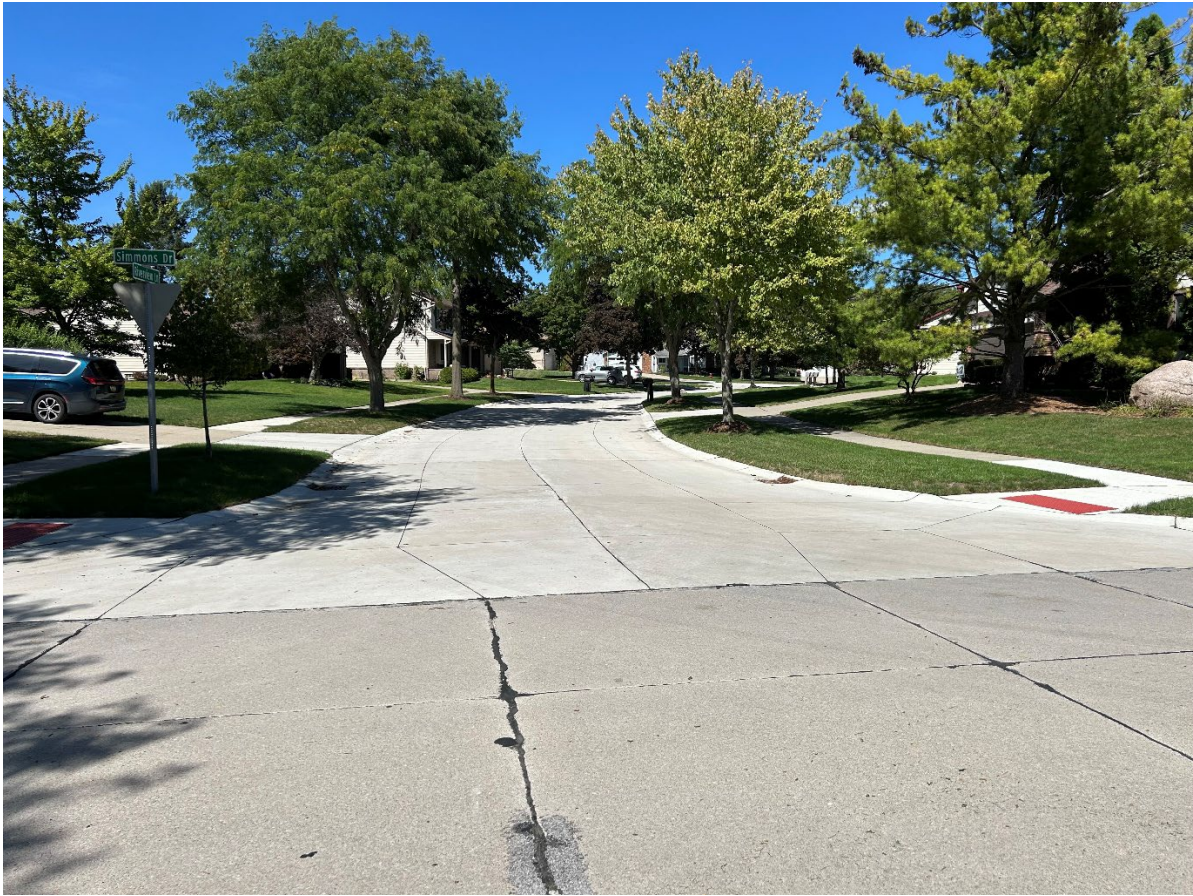
After: Riverview Lane, looking north from Simmons Drive.
