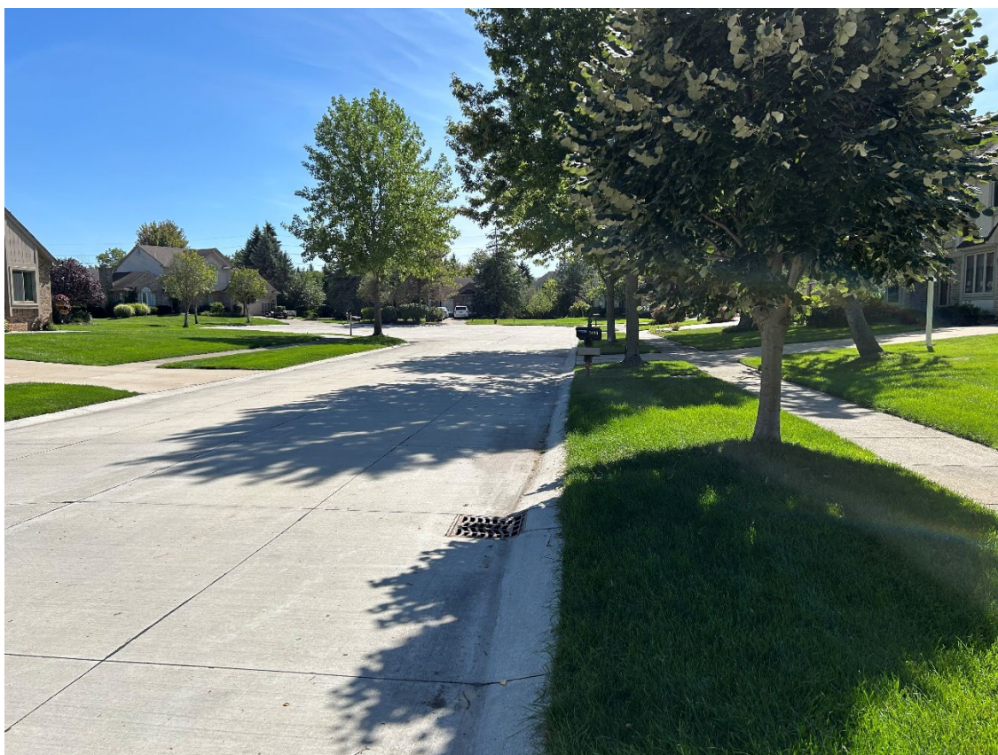
After: Venice Court, Looking south from Roma Ridge Drive.
