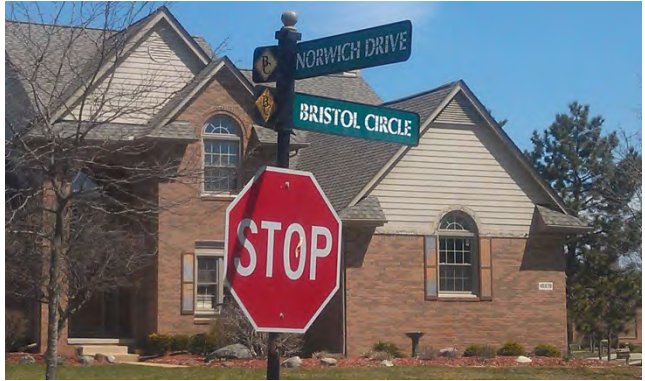
Faded/peeling lettering on street name sign and leaning post.
