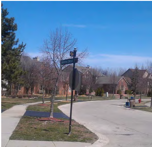
Missing street name sign. Stop sign is rotated almost 90 degrees on the post
