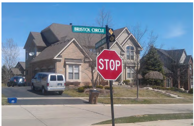
The post is leaning and the street name sign blade is bent.
