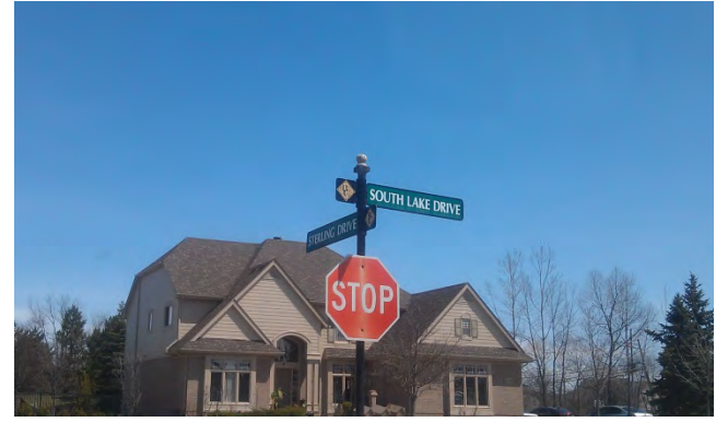
Stop sign is faded and needs to be replaced.
