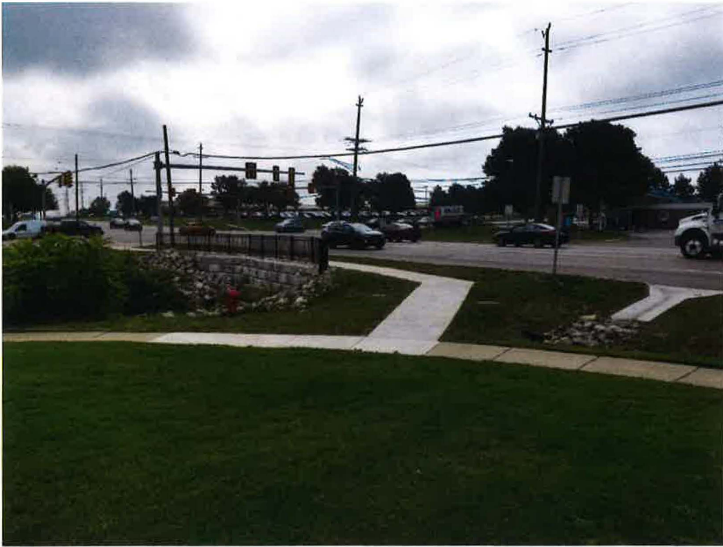
Replaced sidewalk and block retaining wall at Grand River and Haggerty – looking SE
