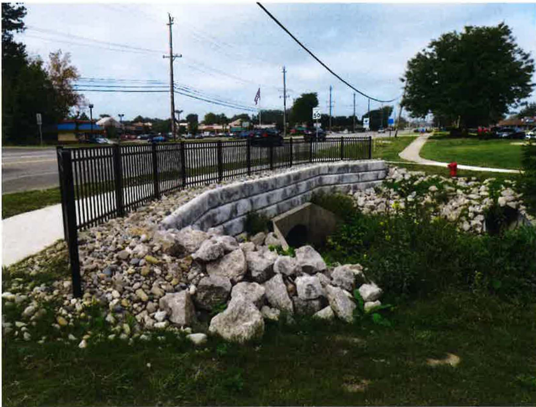
Replaced sidewalk and block retaining wall at GR/Haggerty – Looking southwest
