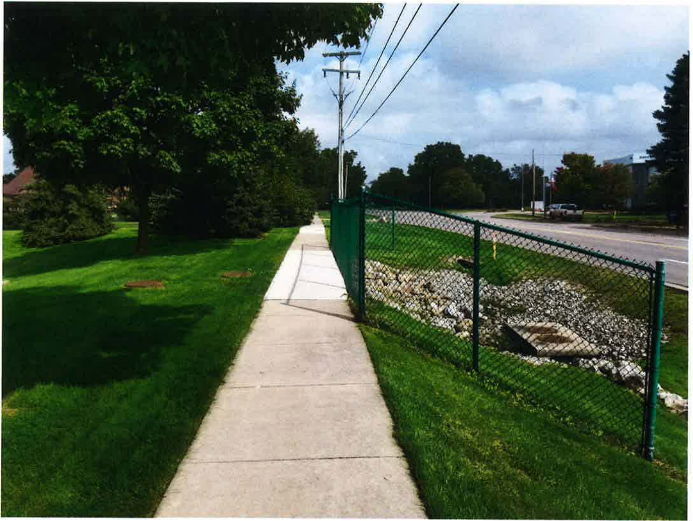
Replaced sidewalk flags and gaps along Haggerty, south of 9 Mile Road.
