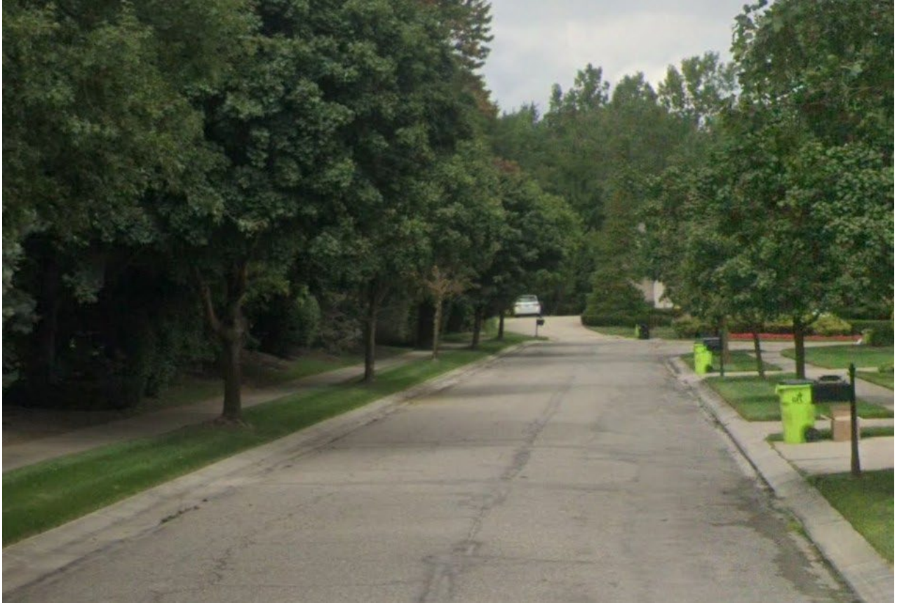
Before: Amberlund Court, looking from Nine Mile Road
