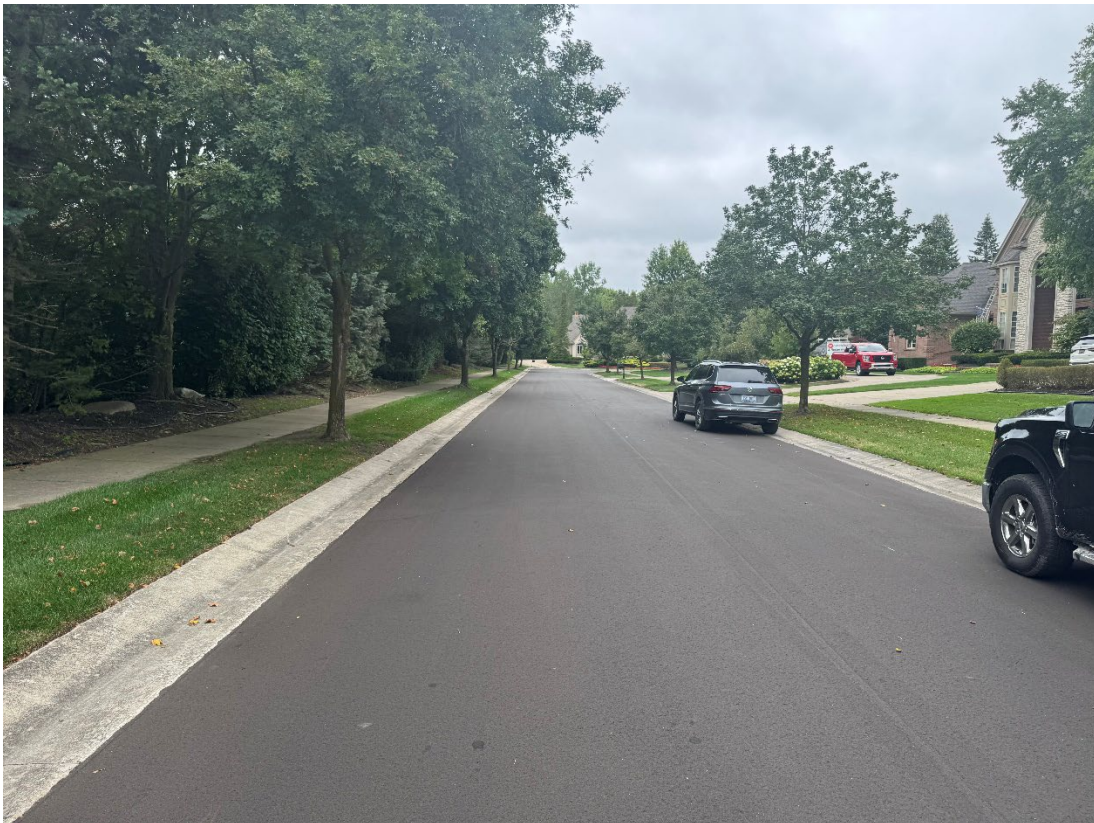
After: Amberlund Court, looking from Nine Mile Road
