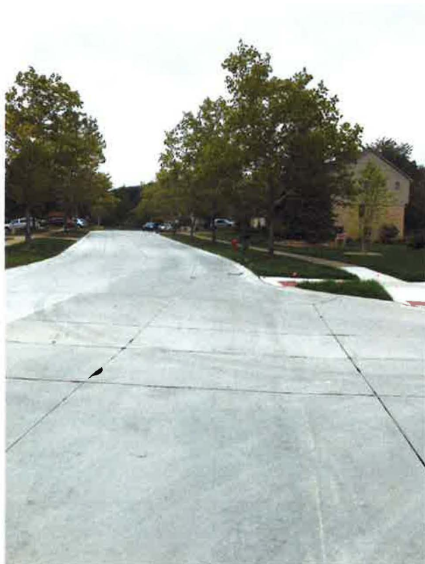
Post-Construction photo example of Moorgate Street, looking north from Havergale Street
