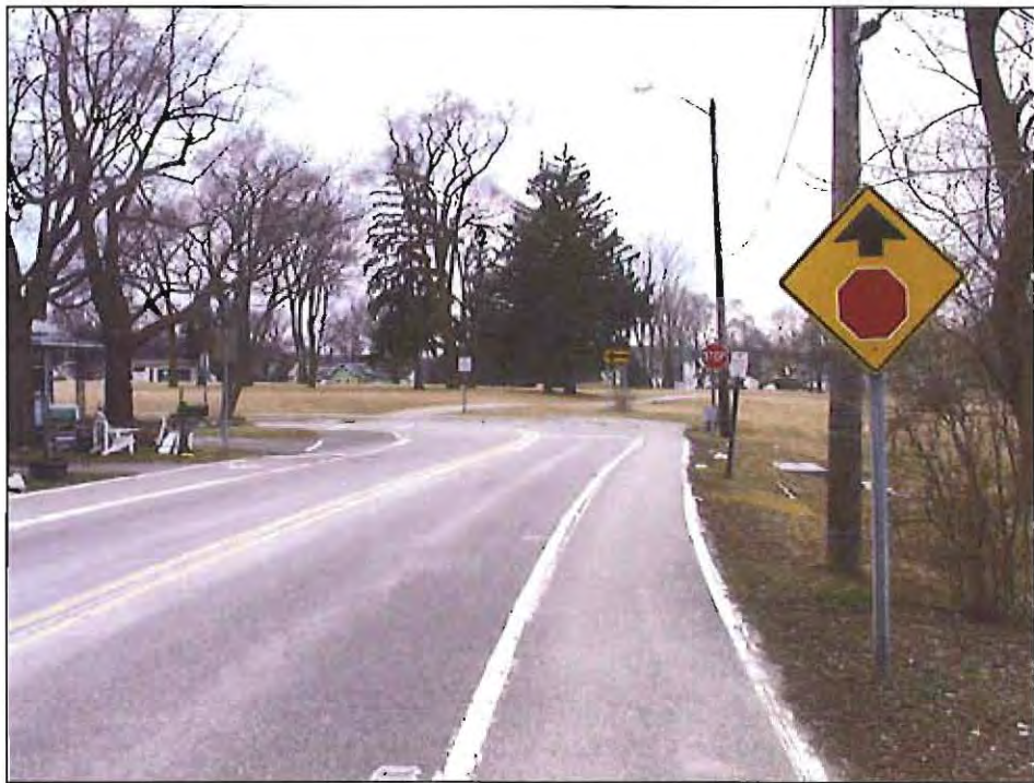
Figure 6. Looking Generally West at Bend in East Lake Drive
