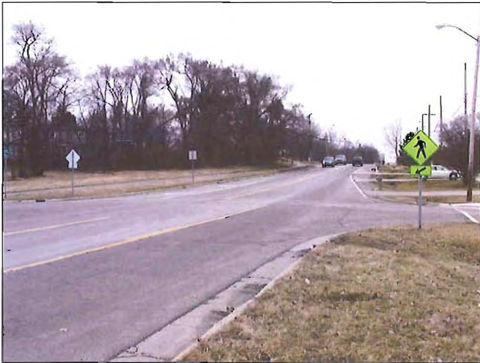
Figure 8. Signing for Crosswalk on 13 Mile Road at East Lake Drive
