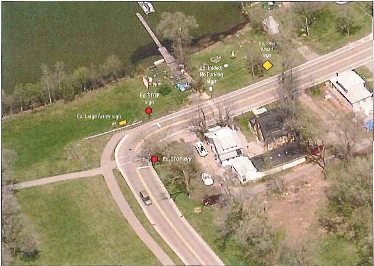
Figure 2. Birdseye View of Bend in East Lake Drive and Existing Traffic Signs
