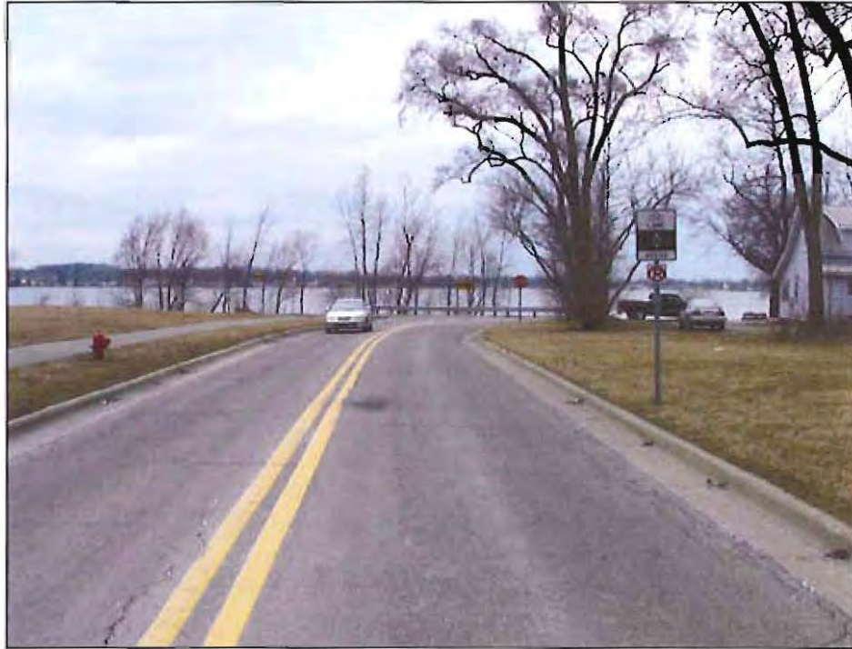
Figure 3. Looking Generally North at Bend in East Lake Drive
