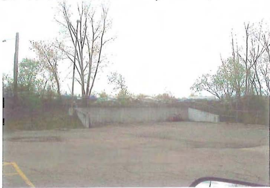
view of storage facility from post office
