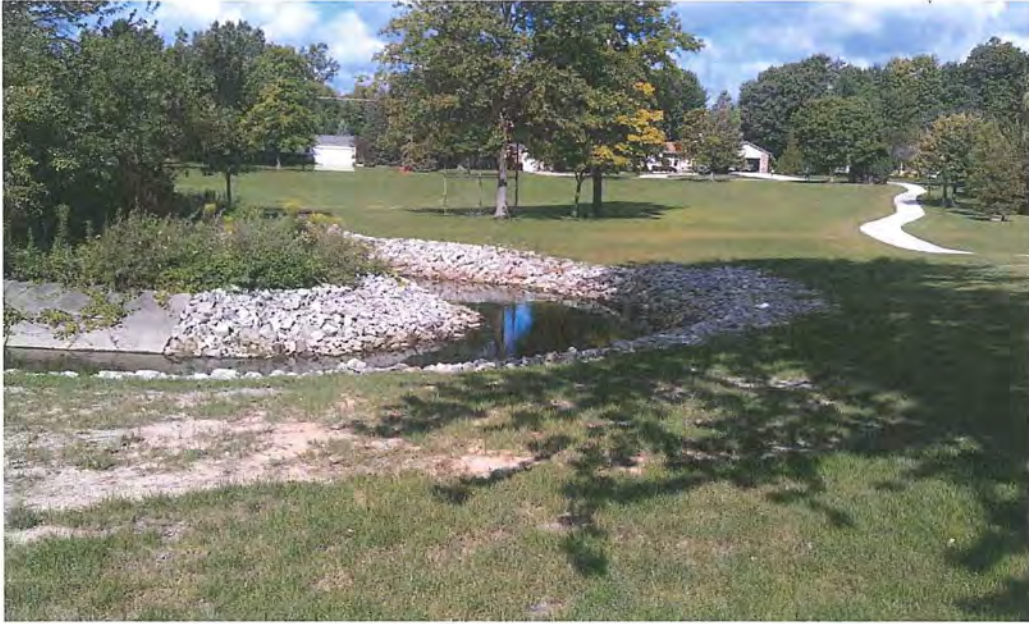
Streambank stabilization along the Rouge River
