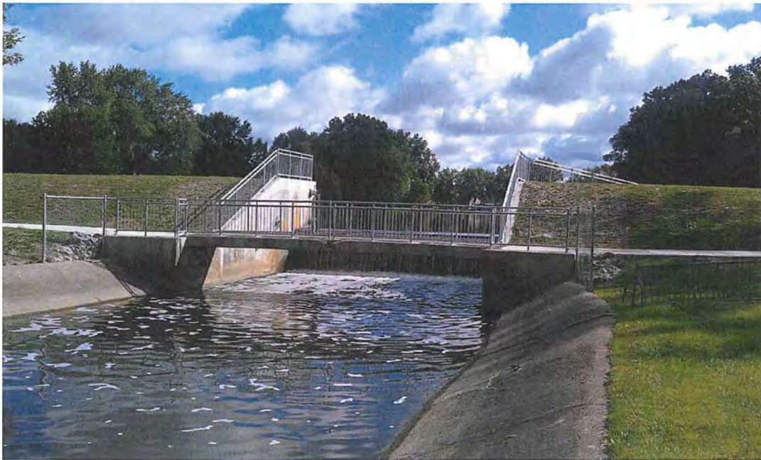
Looking north at the dam
