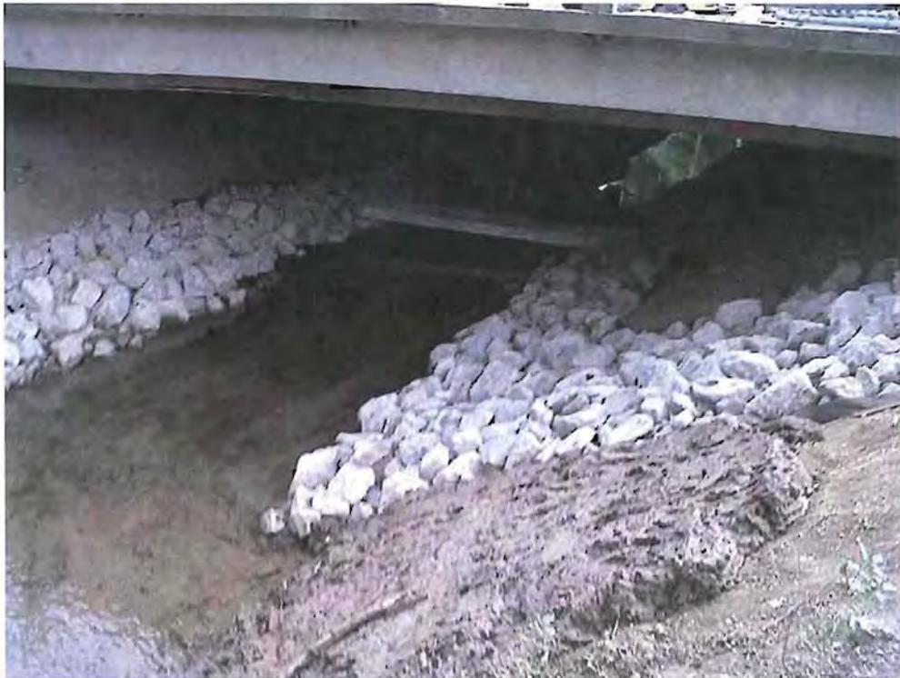
**Underside of Cranbrooke Drive with slope stabilization AFTER**
