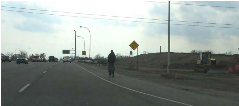
Existing conditions for the Novi Street overpass
