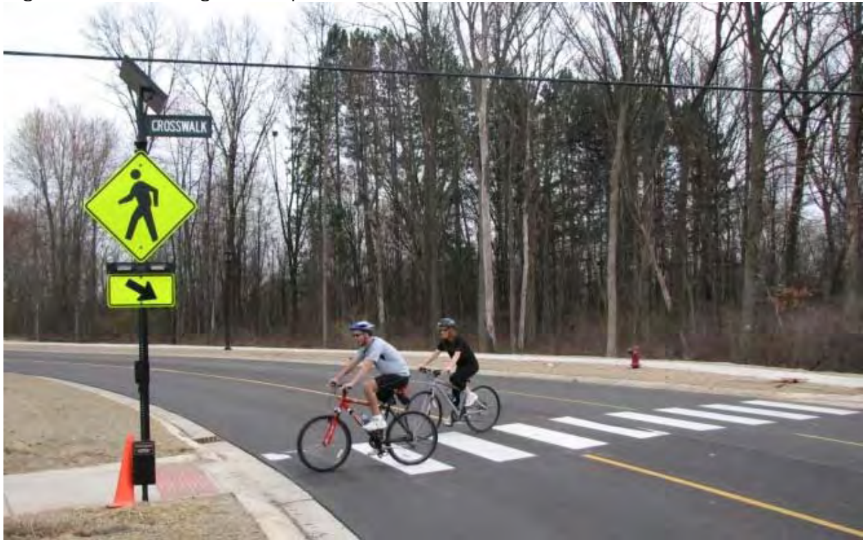
Fig. 5.7H. Rectangular Rapid Flash Beacon
