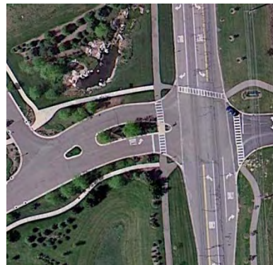
Raised Median at Glenwood Dr Entrance
