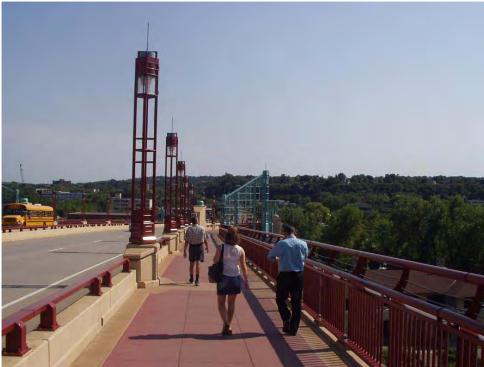
Wabasha Street Bridge in St. Paul Minneapolis
