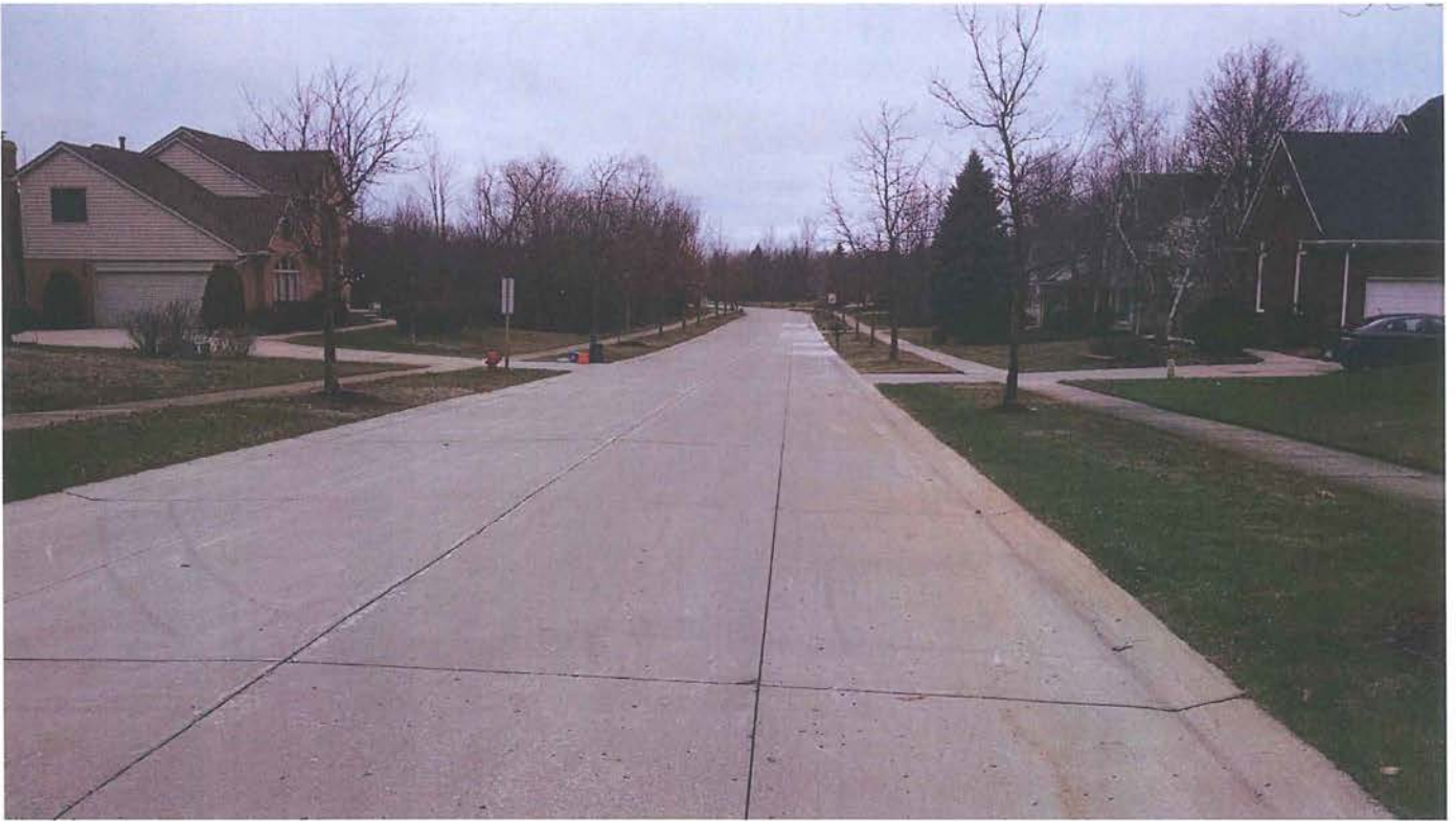
Arcadia Drive – concrete roadway panel replacements (added contract work)
