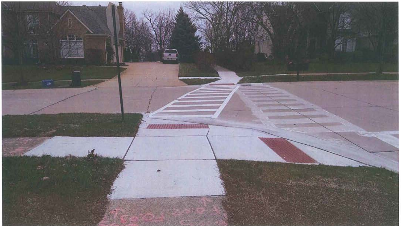
Intersection of Arcadia and Cordoba Drives, ADA sidewalk ramp improvements
