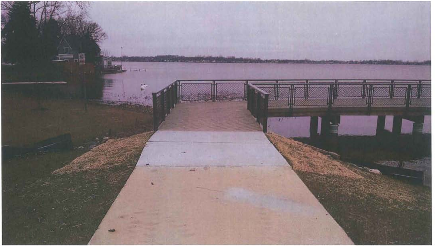
Pavilion Shore Park – West sidewalk/boardwalk transition replacement (added work)
