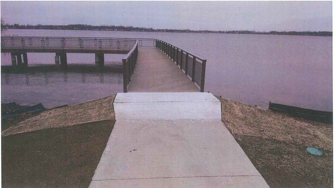
Pavilion Shore Park – East sidewalk/boardwalk transition replacement (added work)
