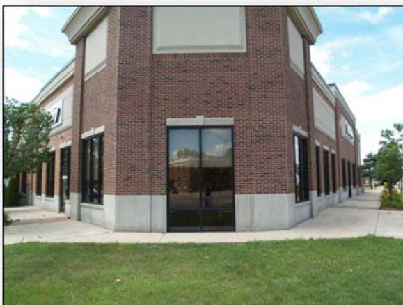
Existing pedestrian-oriented commercial development in the North West Area.
