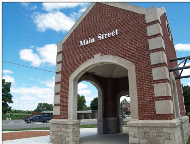
Existing gatehouse structure at Grand River and Main Street.
