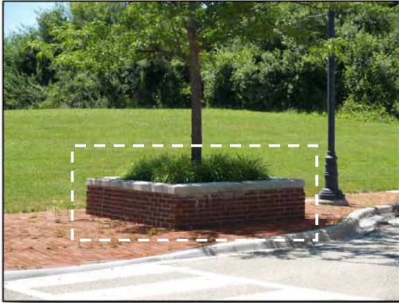
Example of a masonry planter with limestone cap located on Main Street.
