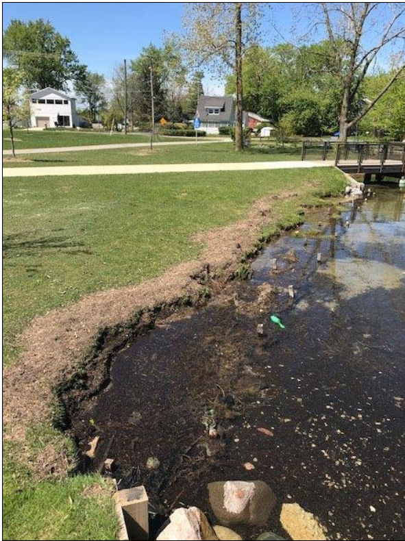
Pavilion Shore facing west (Sept. 2017)
