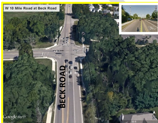
Figure 21. Beck Road at 10 Mile Road
