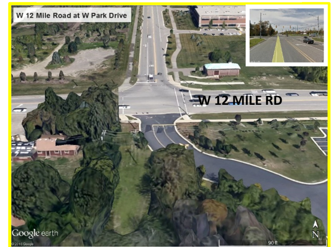
Figure 25. W Park Drive at 12 Mile Road
