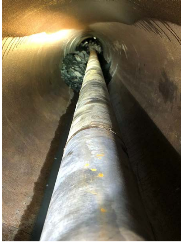
Boring shaft and Hammer-Head bit in a casing pipe
