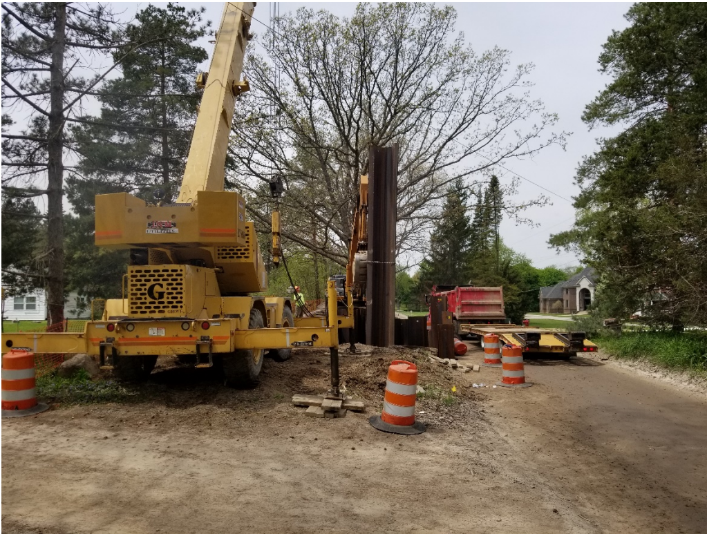
Installing sheet piles for Shaft No. 9
