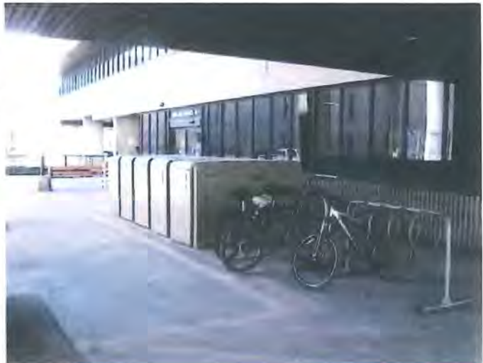
Covered bike parking under roof overhang with bike lockers
