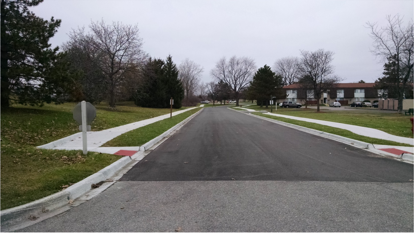
Wedgewood Drive – Looking north from Springlake Boulevard.
