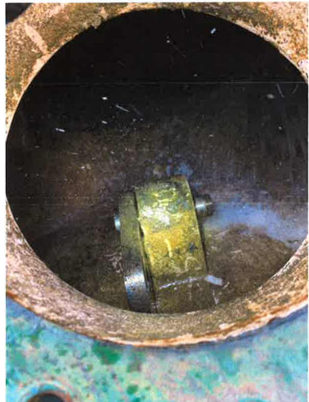
Hydromax USA repairing dashpot assembly on 24" check valve – Houston 2020
