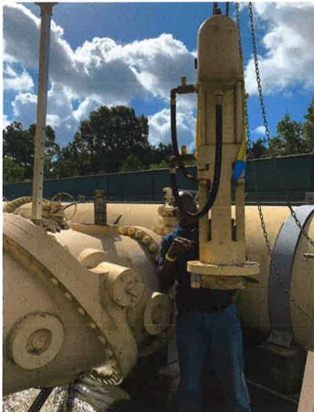
Hydromax USA repairing dashpot assembly on 24" check valve – Houston 2020
