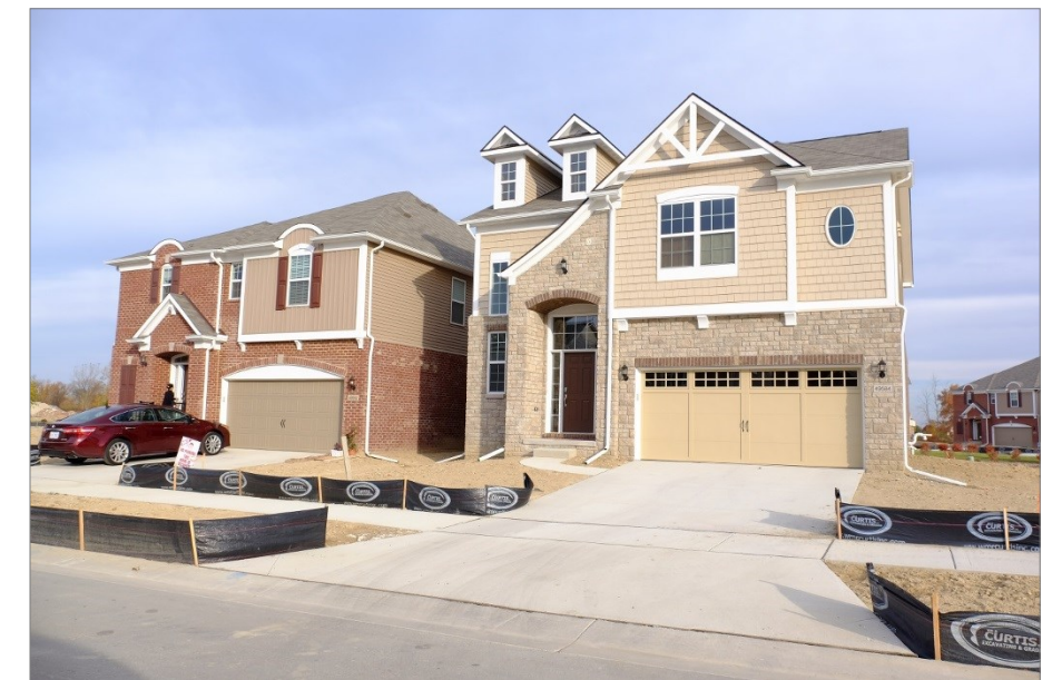
Top: existing pattern of single-family residential subdivision; Bottom: Berkshire Pointe, a more recent residential development with higher density.
