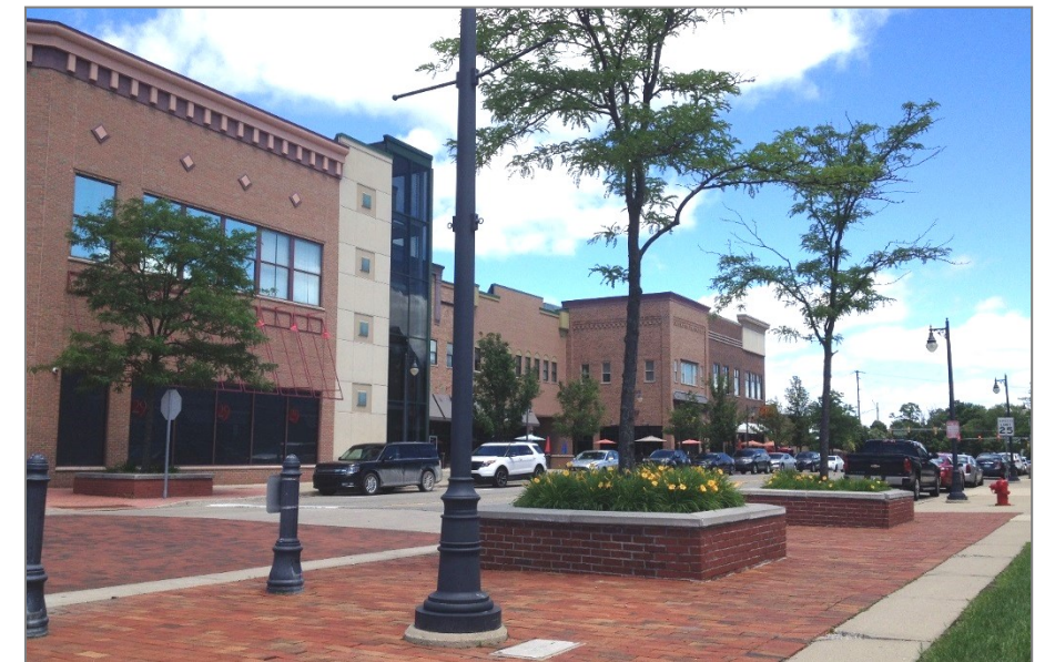
Commercial development in Novi features a range of typologies, including malls (not pictured), large suburban strip centers with parking entirely in front (top), small strip commercial with limited front yard parking (middle), and the Main Street district, which is patterned on more traditional downtown development (bottom). This last approach has recently returned to prominence and will likely continue to grow in the future.
