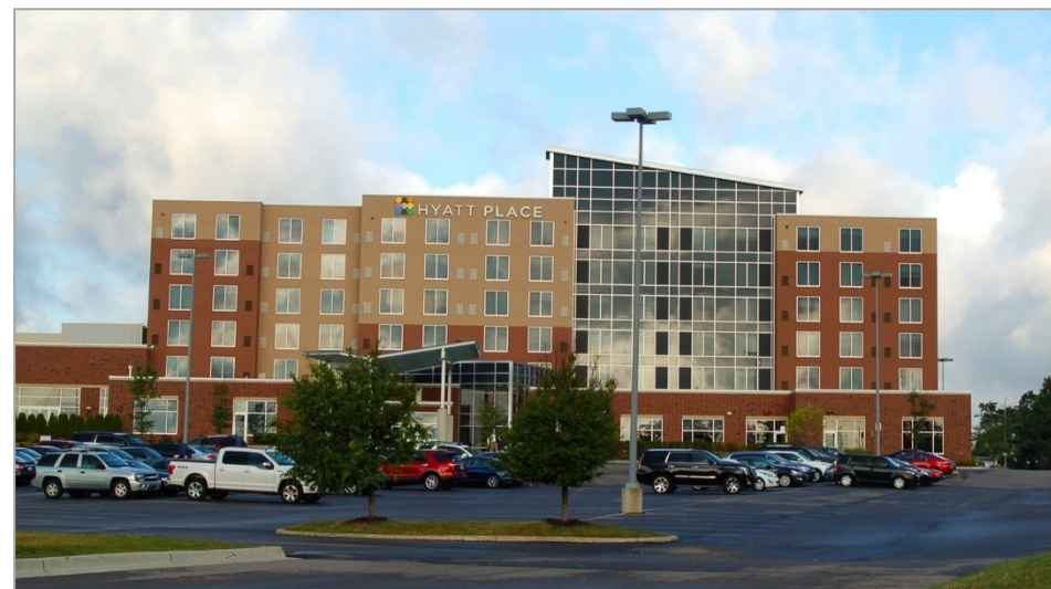
The existing Hyatt Place hotel at the Suburban Collection Showplace is similar in scale and impact on utility service as many of the use options proposed for the interstate-adjacent portion of City West.
