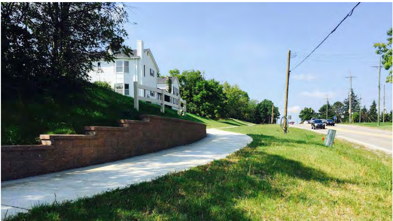
Completion of missing segment 129 connecting Maples of Novi to Haverhill Farms along Fourteen Mile Road
