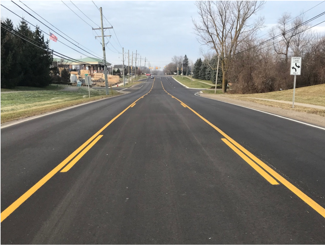
AFTER – Looking west towards Novi Road
