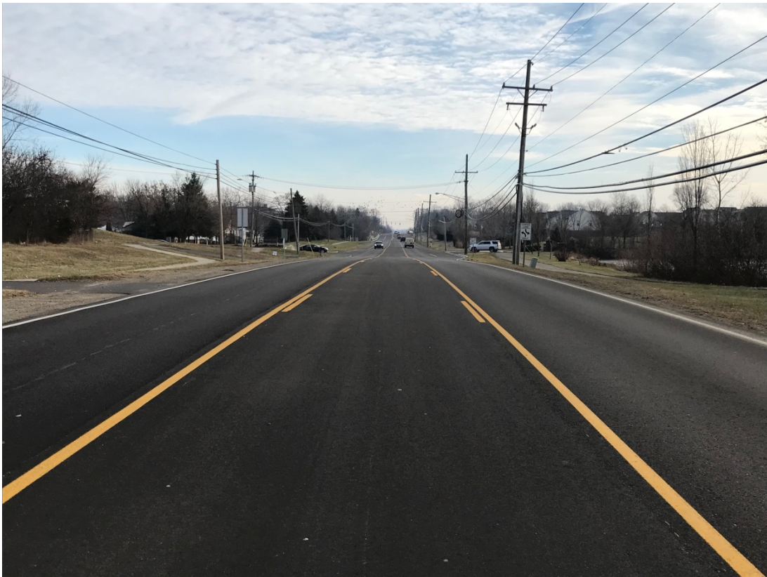
AFTER – Looking east towards Meadowbrook Road
