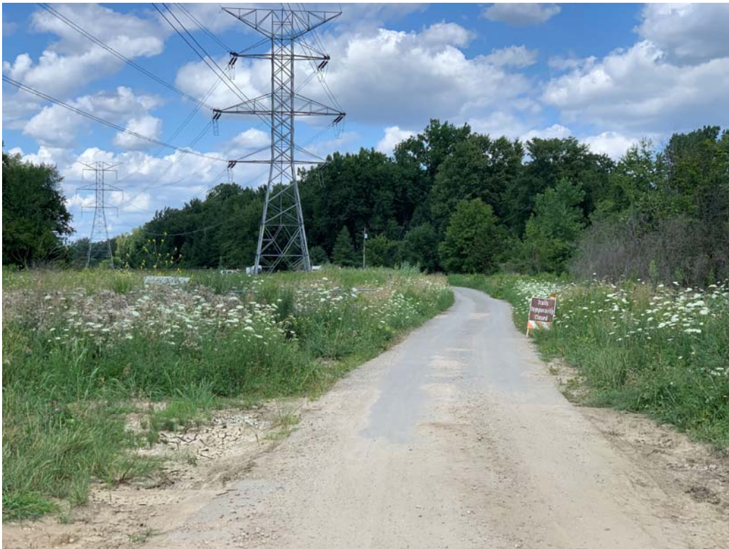
Under Construction: ITC Trail between Nine Mile Road and Ten Mile Road
