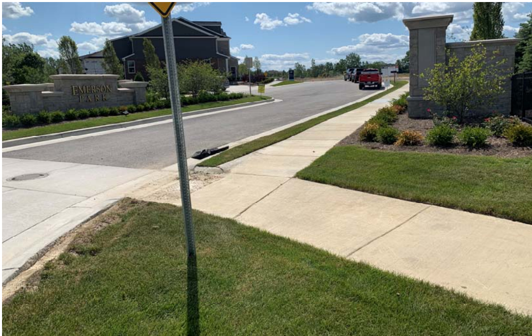
Existing sidewalk widened to 6 feet as part of Private Development along Novi Road
