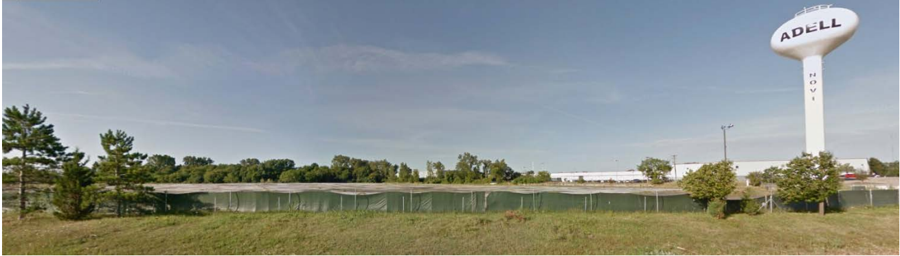
Existing Streetscape along I-96 frontage
