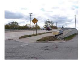
12 The bridge offers gateway opportunities and needs enhancement
