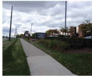
14 Lack of street trees to help separate pedestrians from traffic lanes
