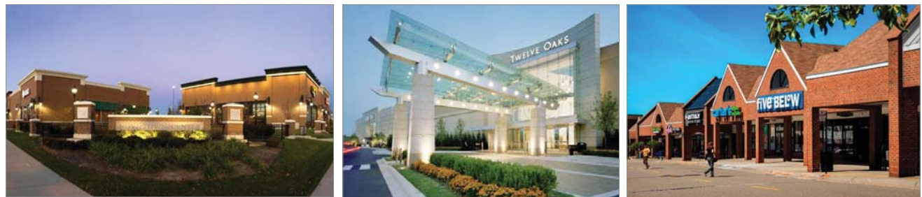
Photos above from the Novi Town Center (left), Twelve Oaks (center), and West Oaks II (right)
