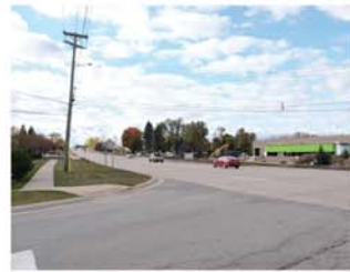
10 The corridor lacks amenities such as pedestrian lighting
