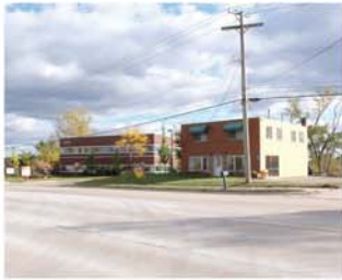
9 The corridor lacks unifying characteristics
