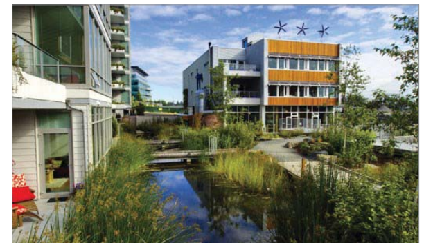
The images above illustrate examples of mixed use development that incorporate water features into the site in ways that create attractive spaces that also assist with stormwater development. From top: Discovery Green (by DiscoveryGreen.com), the Avenue (by Sasaki), and Dockside Green in Victoria, BC (DocksideGreenSales.com)
