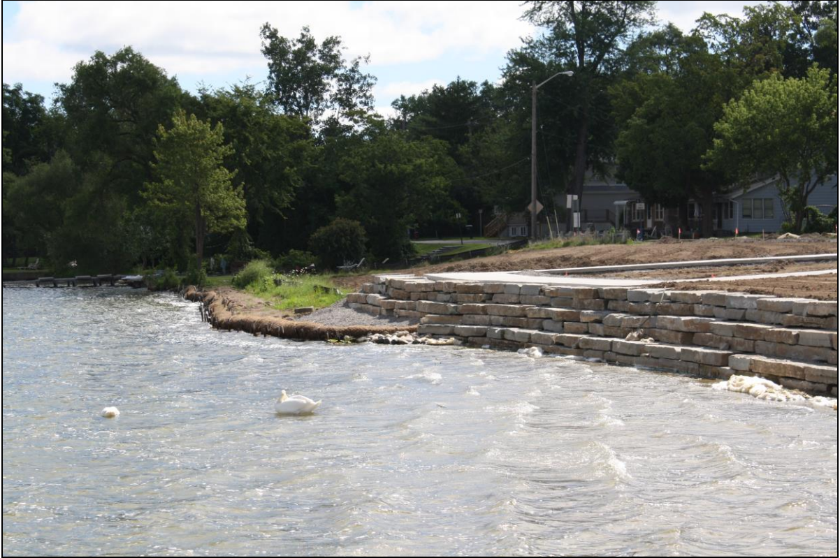
Pavilion Shore facing east (July 2013)
